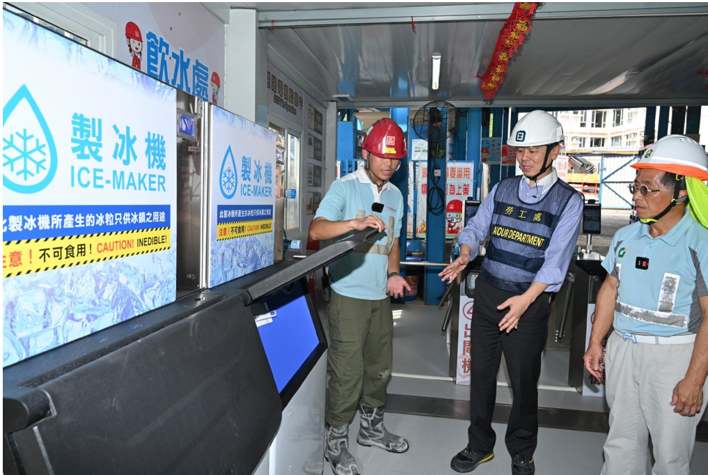
Mr. Vincent FUNG, Acting Commissioner for Labour (centre), and Ir Thomas HO, Chairman of the Construction Industry Council (1st right), having a look at the ice-maker at the construction site
