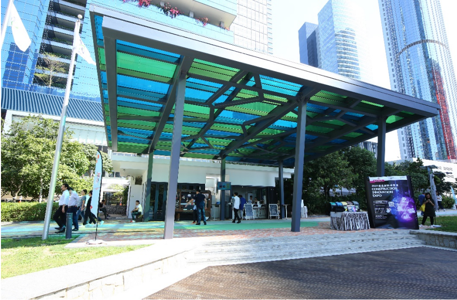
The Air Improvement Photovoltaic (AIPV) Glass Canopy
