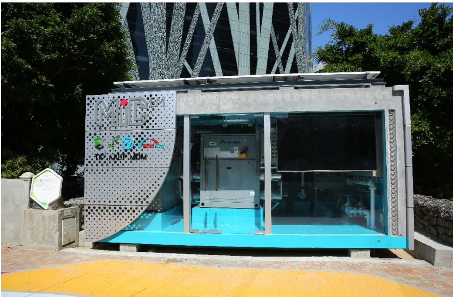
Dedicated to advancing green facilities, the CIC-ZCP has introduced Hong Kong's first Electrical and Mechanical Modular Integrated Construction (emMiC) for Stormwater Cooling System
