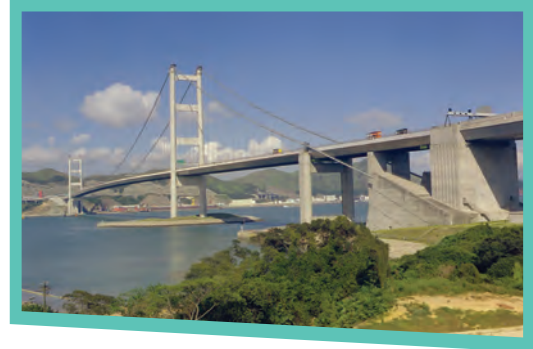
Bridges and Tunnels
