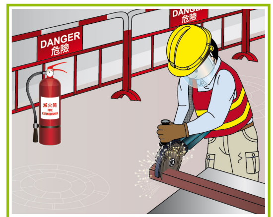
Provide fire extinguishing equipment
