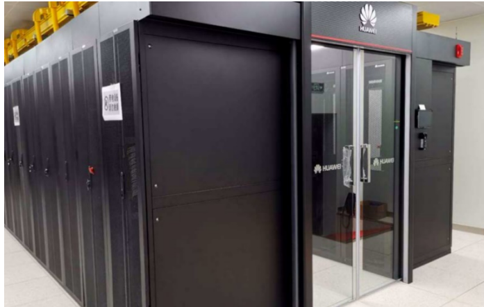
Figure 8.4 IT rack module, which integrates in-row cooling, Uninterruptible Power Supply (UPS) and the aisle containment (Photo courtesy of BYME Engineering (H.K.) Limited)
