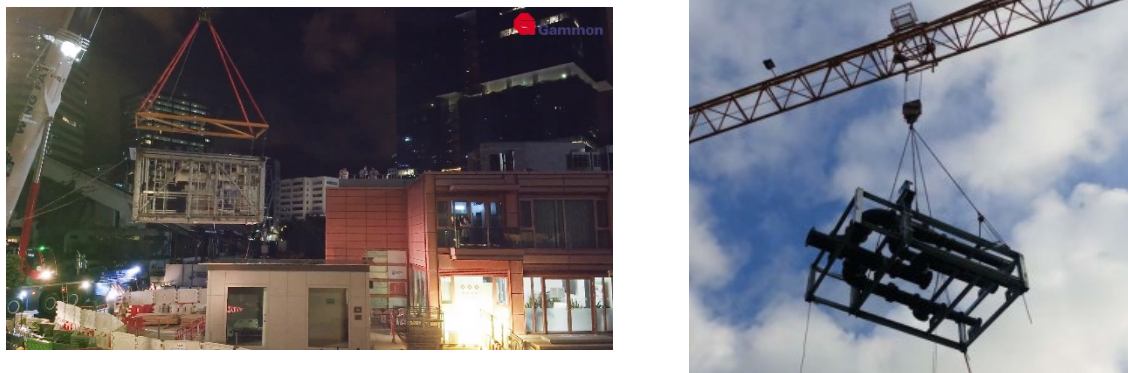
(a) Lifting of MEP service module by mobile crane (Photo courtesy of Gammon Construction Limited) (b) Lifting of pipe module by tower crane (Photo courtesy of FSE Engineering Group Ltd.)
