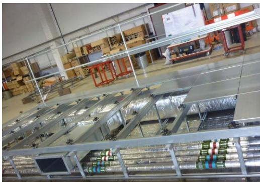
(a) Horizontal MEP modules with false ceiling panels and frames
