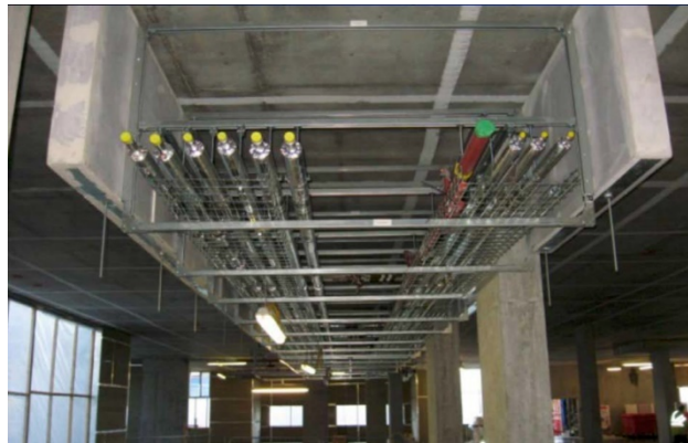
Figure 6.3 Horizontal module integrated with partition wall (Courtesy of BYME Engineering (H.K.) Ltd.)
