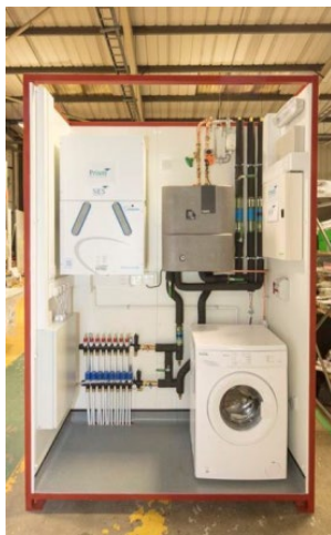
(a) Utility cupboard completed with underfloor heating components with a washing machine etc.
