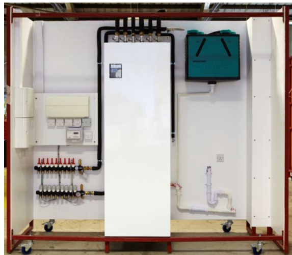
(b) Utility cupboard completed with electrical installations and underfloor heating components etc.
