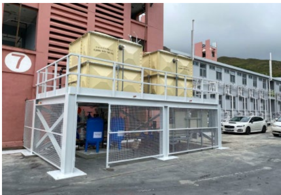
(a) Pump room modules
