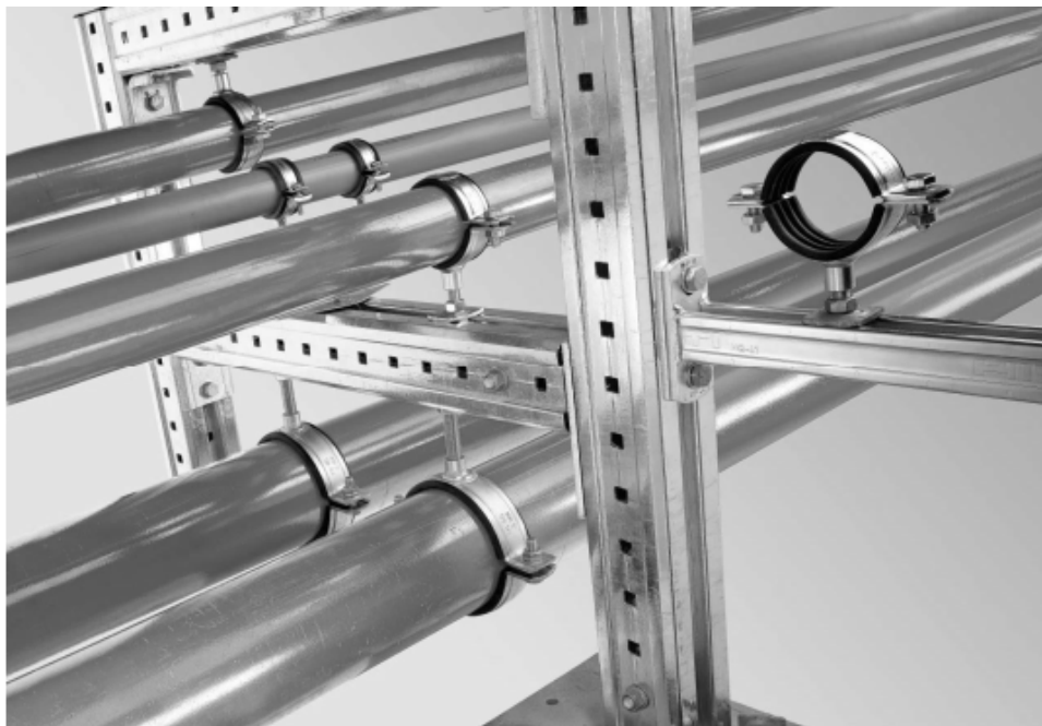
Figure 4.2 Access space provided between vertical tiers within a module (Courtesy of Hilti)
