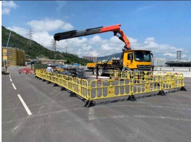
Photo 2 Use of mobile crane in delivering pipe modules
