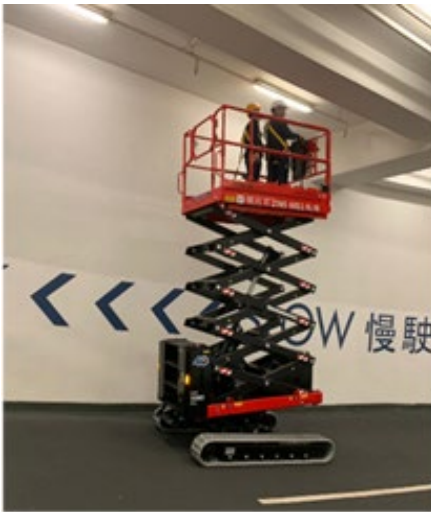
(c) Working platform working on sloped terrain
