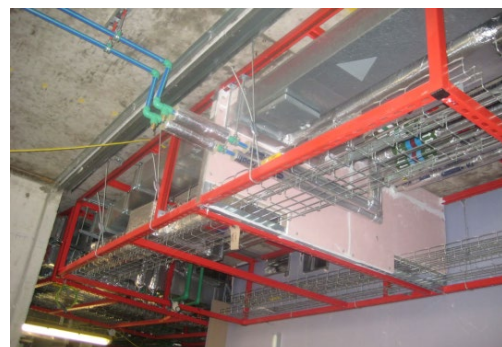
(b) Horizontal MEP modules completed with Firestop board
