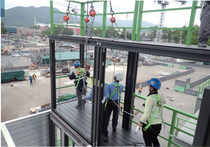
■ Students taking the “Modular Integrated Construction (MiC) Unit Safe Installation” commissioned course at Tai Po Training Ground
