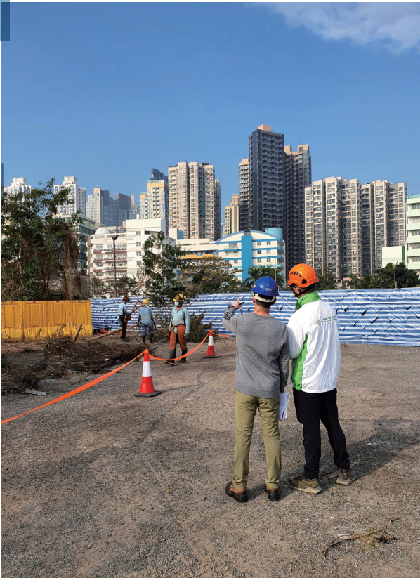
■ Training tutor and arborist trainee were supervising tree removal work by the chainsaw operator at construction site
