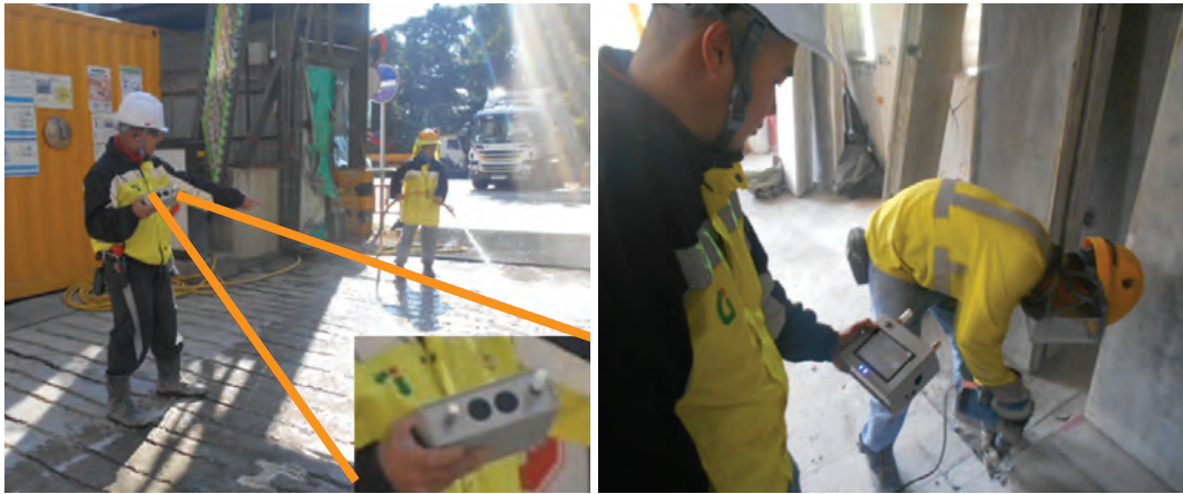
Figure 22 Real-time mobile monitoring of the construction site and immediate action to reduce the pollutants
