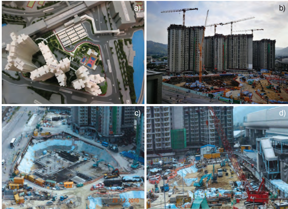
Figure 32 Different stages and parts of the construction site (a) Complete model of the Hip Hing Construction site; (b) Early stage of the Ping Yan Court; (c) Commercial Centre & HOS Run In Out; (d) Public Transport Interchange (PTI) of the site
