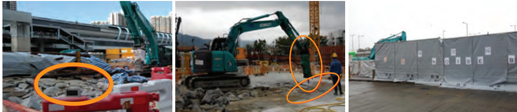
Figure 27 Application of muffler and sound insulation fabric at the concrete breaking area
