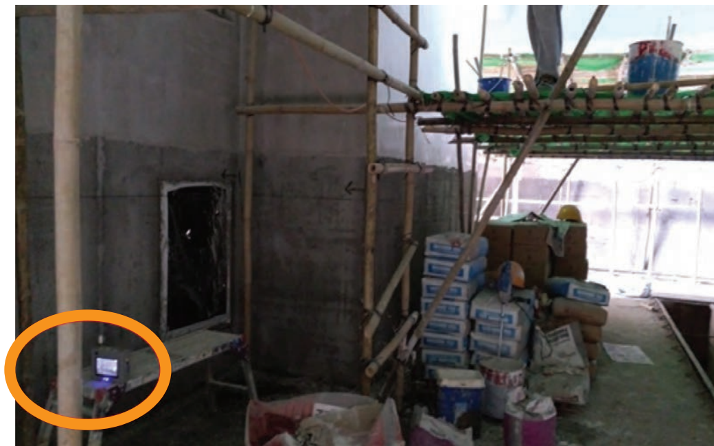
Figure 29 Monitoring indoor paintings to measure abnormal VOC level
