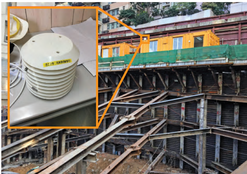
Figure 19 Installation of IEMD in the construction site on MacDonnell Road
