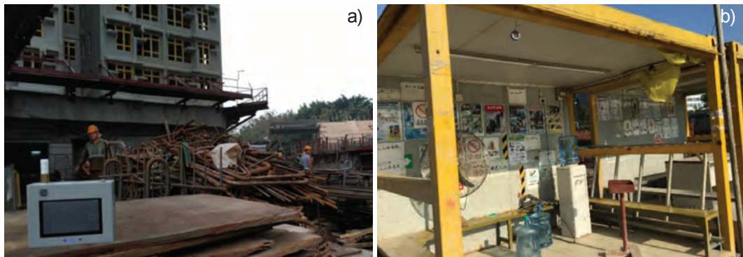
Figure 26 Operational use of IEMS in the bar bending yard. (a) Monitoring by the IEMD; (b) Shelter area for extreme conditions
