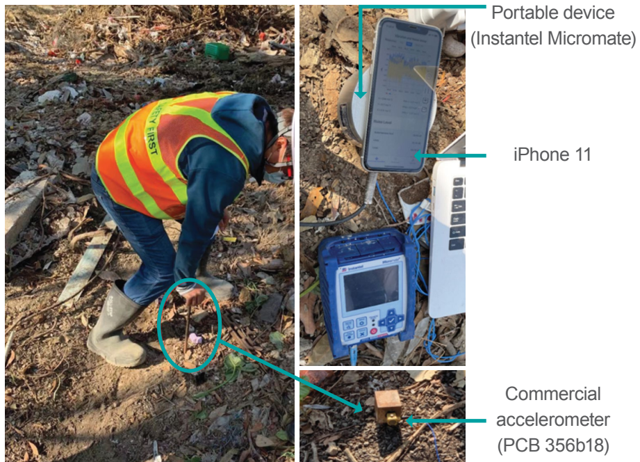
Figure 14 Installation of soil nail, portable vibrometer, iPhone 11, and traditional accelerometer
