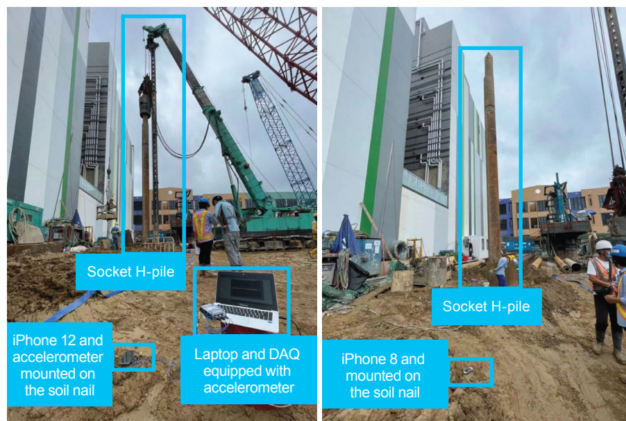
(a) Installation of iPhone 12, tradition accelerometer, and soil nail (b) Installation of iPhone 8 and soil nail
