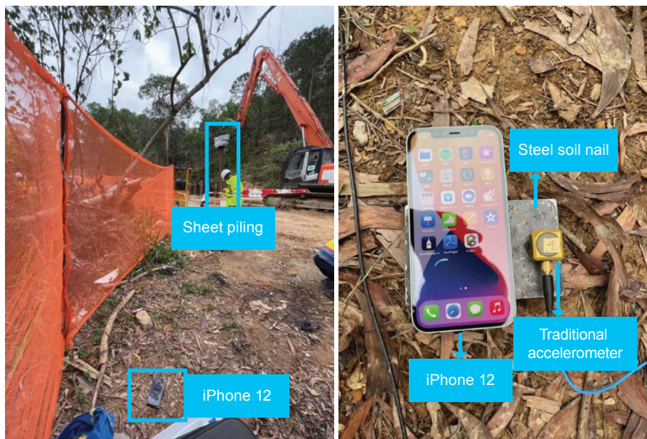
(c) Measurement location of iPhone 12 (d) The installation of iPhone 12, traditional accelerometer, and steel soil nail
