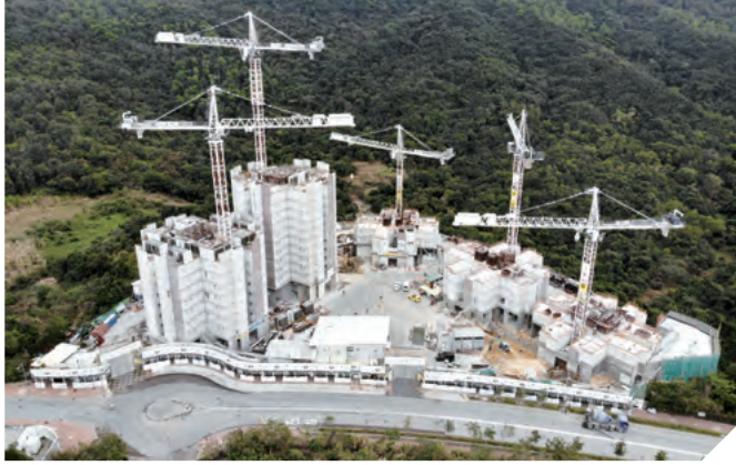
Construction progress at the Disciplined Services Quarters for the Fire Services Department at Pak Shing Kok, Tseung Kwan O
