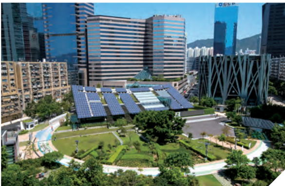
Renovation works phase I were completed in 2019 建造業零碳天地第一階段翻新工程於2019年完成
