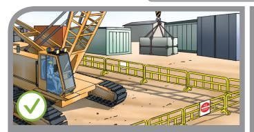
Properly fence the lifting zone with barricades and demarcate with prominent notices and ensure no persons (other than the crane operator) stay within the zone during the lifting operation.
