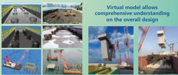
Digital twin for the design of precast V-piers
