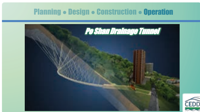
Po Shan Drainage Tunnel
