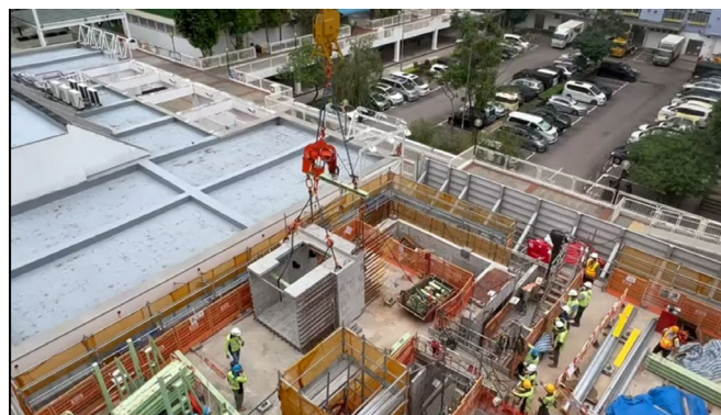
將MiC Lift Core原地吊運豎直 (短片示範)
