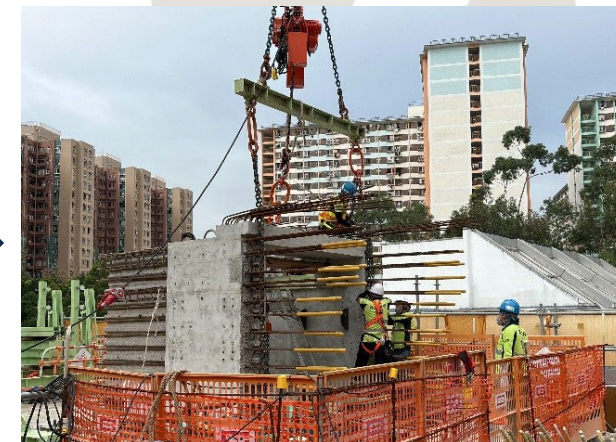
吊運團隊加設吊具準備將MiC Lift Core原地吊運至豎直
