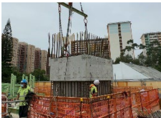
MiC Lift Core原地吊運至豎直
