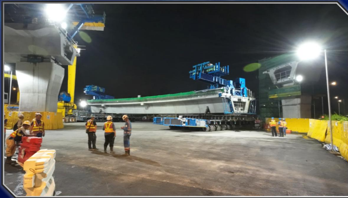
Trial run across Fanling Highway
