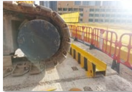
Install Crane Kicker near the Retaining Wall 在擋土牆附近的起重機安裝阻擋設備
