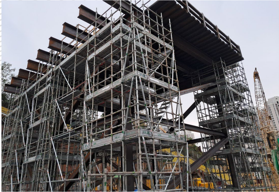
Scaffold Working Platform for Assembly of Steel Platform 金屬棚架工作平台組裝大型臨時鐵台
