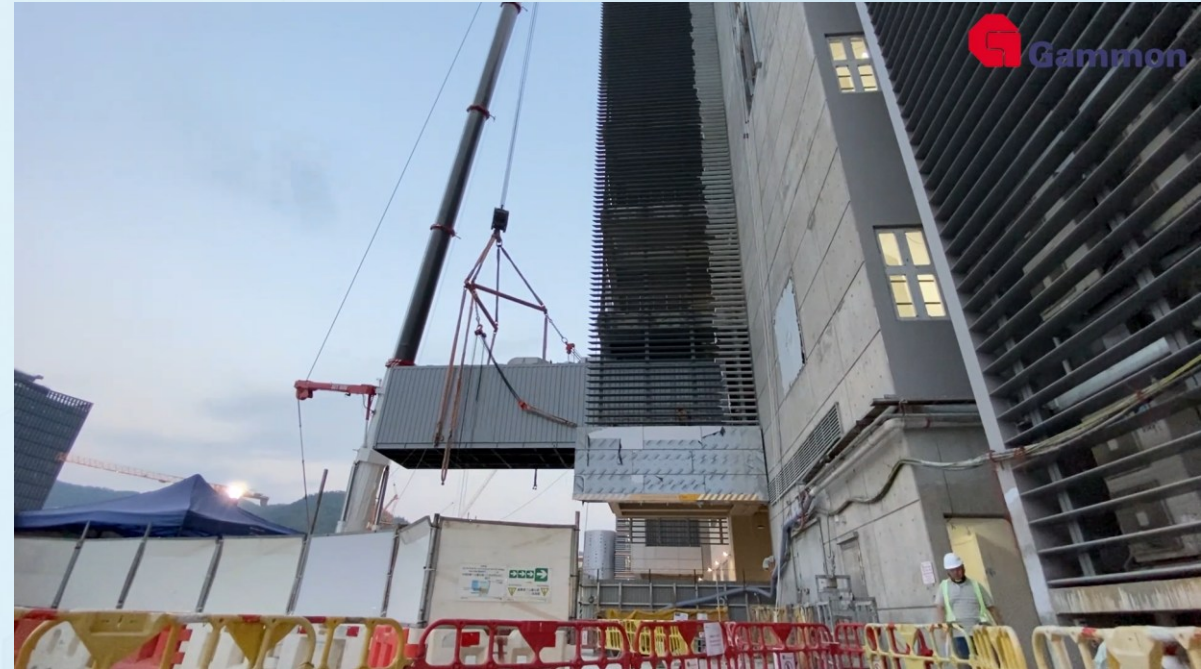
Container Type Gen-set at Phase2
