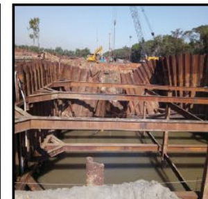
Failure on Cofferdam Construction (Photo Source from internet)
