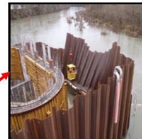
Failure on Cofferdam Construction (Photo Source from internet)
