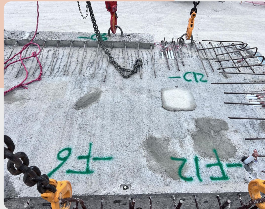
Lifting points marked on MiC Module
