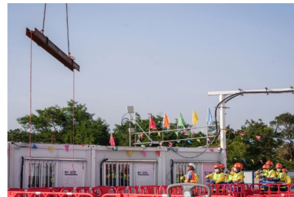
MiC 組裝合成模組/工料吊運練習 MiC / Material Lifting Practice
