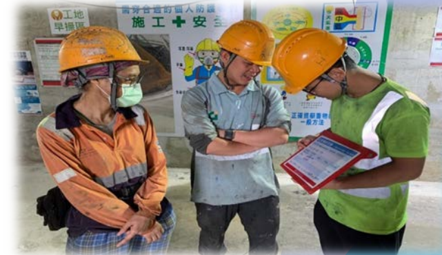
PPE checking & HIA
