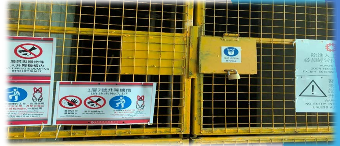
Safety warning signage are posted on lift shaft door and the door is kept locked at all times
