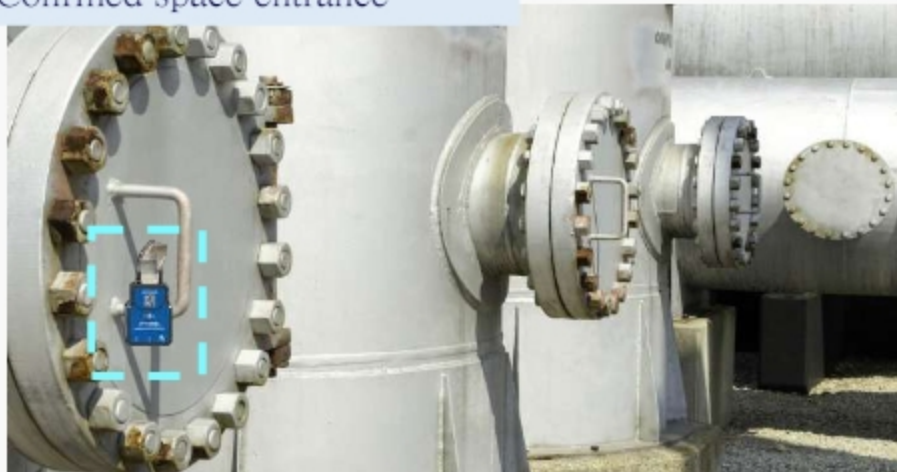
Confined space entrance
