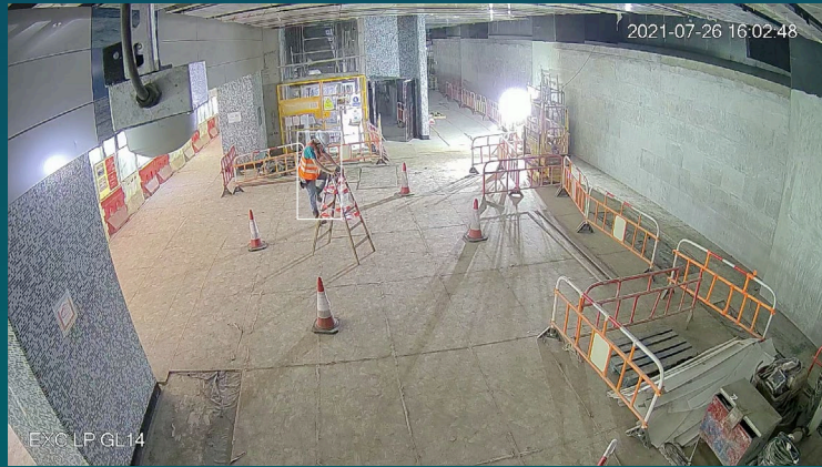
(1) Worker climb up ladder
