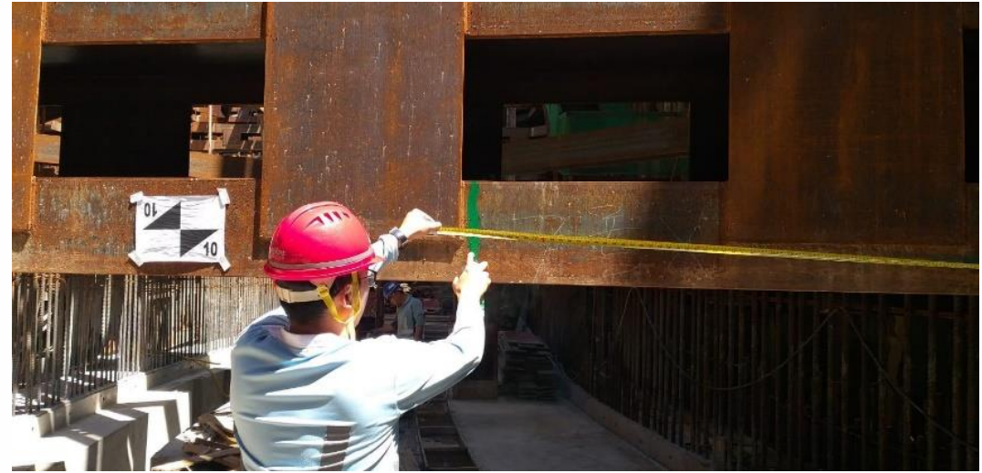
Identify the positions to be cut on strut
