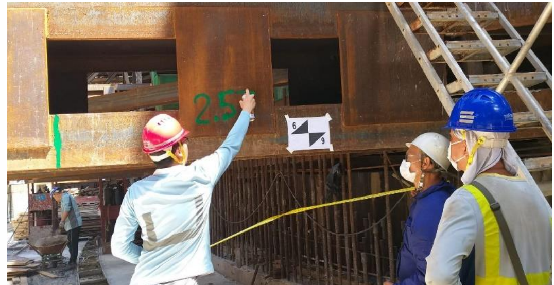
Mark the Weight on the strut
