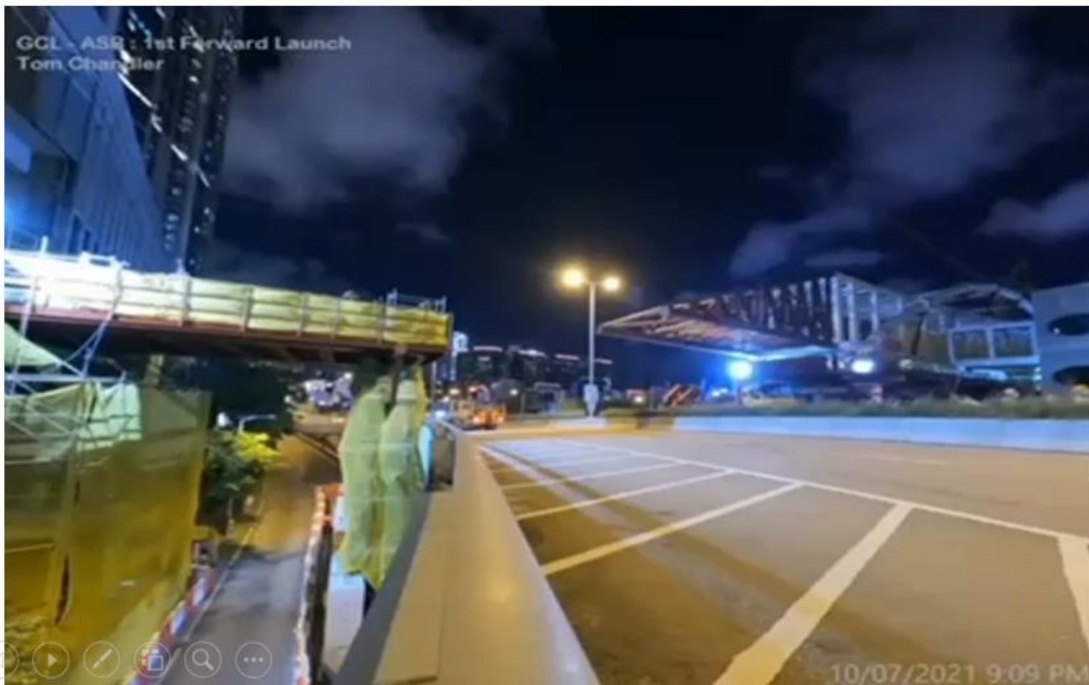
3 Segments for Linkbridge Installation
