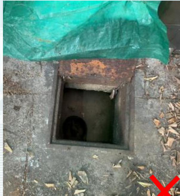
Manhole before sealing
