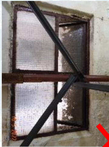
Glazed sashes not yet removed
