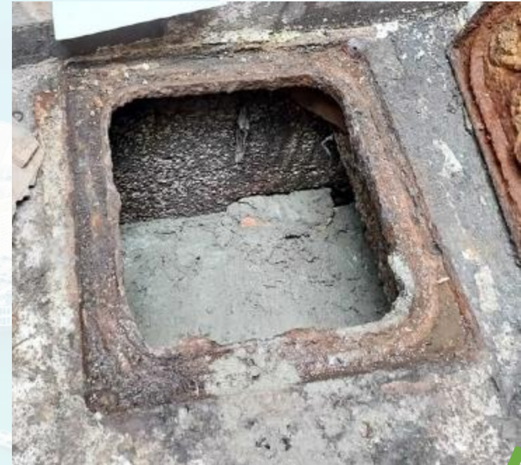
Manhole after sealing
