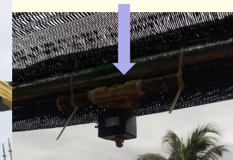
Electric valve receive signal from Electric signal controller
