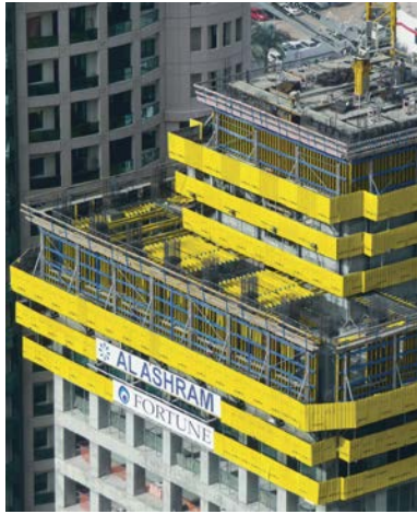
Figure 0-4: Automatic climbing formwork SKE50 plus (Image: Doka GmbH)
