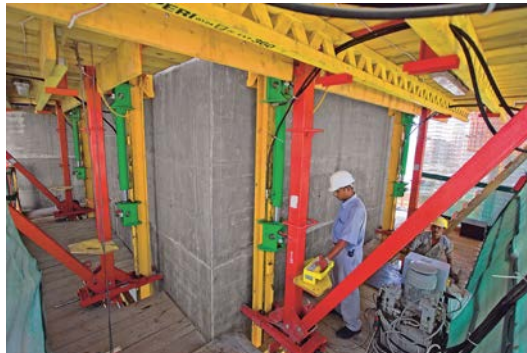
Figure 0-6: The PERI climbing mechanism (Image: PERI GmbH, Weissenhorn)
