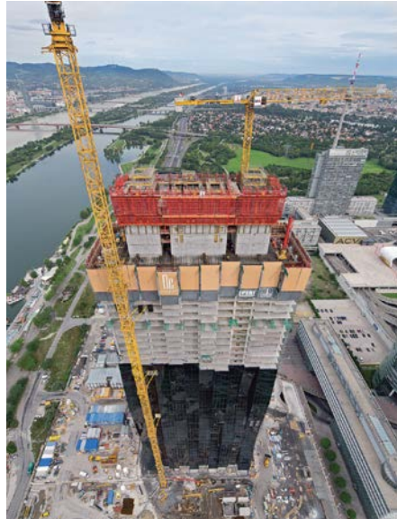
Figure 0-7: ACS in action: The three core areas of the DC tower were moved up independently of each other using an ACS climbing formwork up to a height of 220 m. A 3.50-m concreting section was realized by the construction team in 4 days. (Image: PERI GmbH, Weissenhorn)
