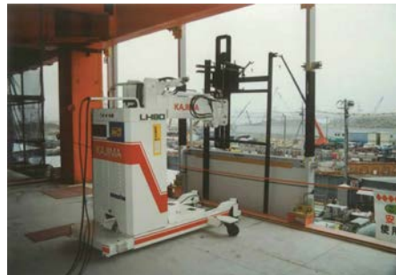
Figure 0-25: Facade element installation robot system operated on the finished floor (Image: Kajima Corporation)
