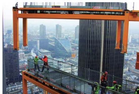
Figure 0-46: Installation of the prefabricated steel table (Image: www.designcurial.com , 2017)
