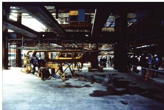
Figure 0-9: Takenaka's horizontal concrete distribution robot in action
