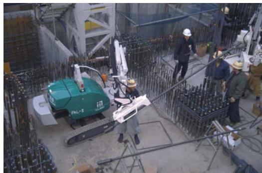
Figure 0-2: Robot for positioning and installation of medium-weight reinforcing bars (Image: Kajima Corporation)
