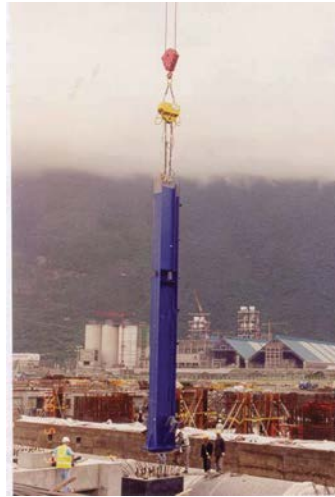
Figure 0-20: Auto-shackle system in action (Image: Samsung and Kwangwoon University)
