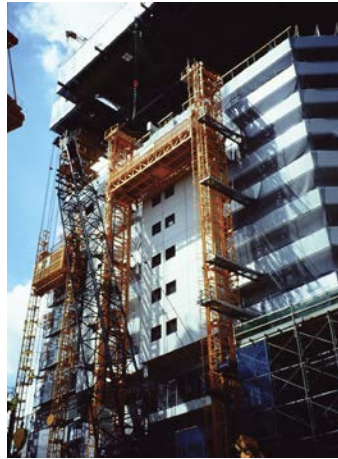
Figure 0-35: Automatic vertical lift (Obayashi Corporation)
