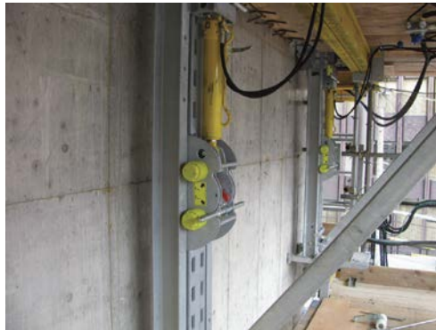
Figure 0-5: Hydraulic climbing mechanism (Image: Doka GmbH)
