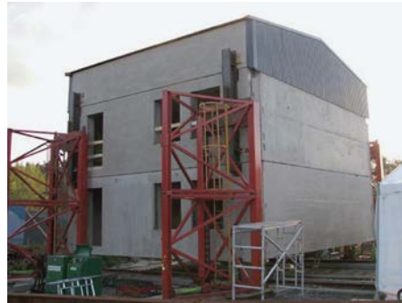
Figure 0-50: Lifting after assembly of ground floor (Image: Skanska)
