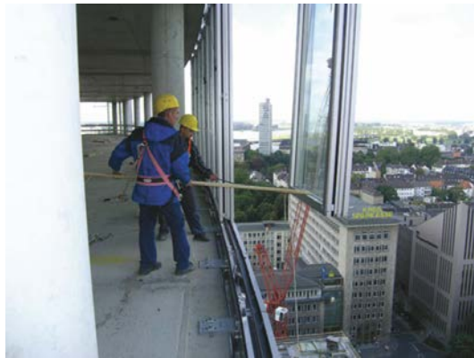
Figure 0-40: Conventional glazing curtain wall installation (Image: www.halfen.com , 2017)
