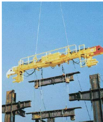
Figure 0-39: Mighty Jack system in action
