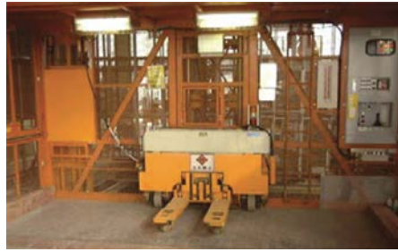
Figure 0-17: The automatic transfer equipment is an intermediary system that can both take up material from a dedicated location in front of a vertical lift to which the AGF has delivered material and unload a vertical lift (Image: Obayashi Corporation)
