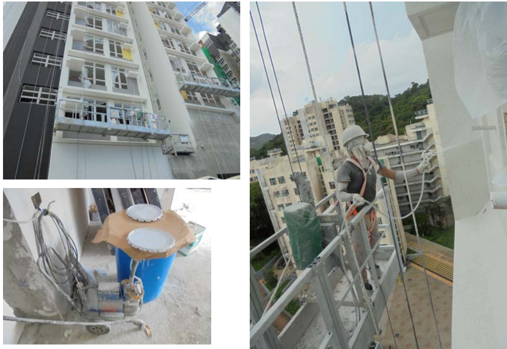
Figure 3-16: Exterior painting application
