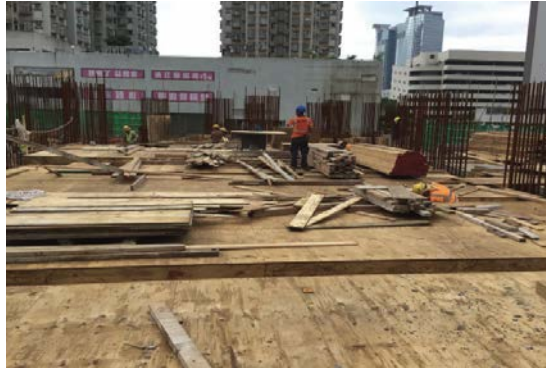
Figure 0-3: Conventional formwork erection on-site. (Image: Hip Hing Engineering Co., Ltd, 2017)
