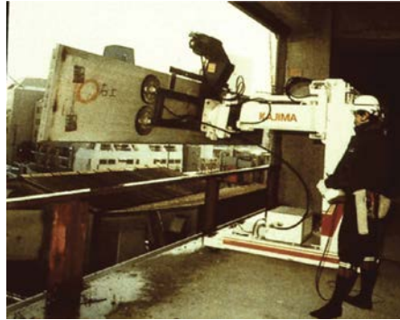
Figure 0-26: Facade concrete panel installation robot, installing facade panel (Image: Kajima Corporation)
