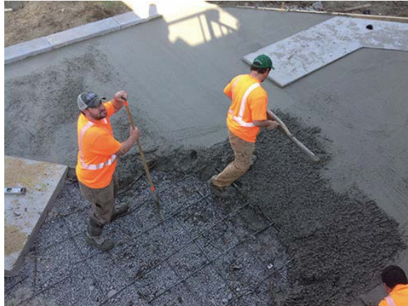
Figure 0-12: Conventional concrete leveling on-site (Image: www.impressionsconcreteandinterlock.com )
