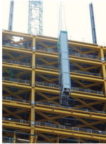
Figure 0-47: On-site assembly of the prefabricated HVAC system (Image: www.ctbuh.org , 2017)
