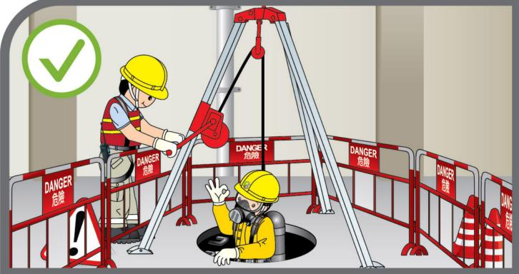
Workers should use suitable safety harness connected to a lifeline that is strong enough to enable him to be pulled out, and that the free end is held by a person staying outside the confined space who has sufficient physical strength to be capable of pulling the worker out of the confined space in an emergency. That person must station outside the confined space throughout the course of work.
