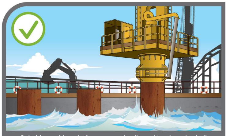
Suitable working platforms, guard-rails and toe-boards shall be provided to machinery used over water.
