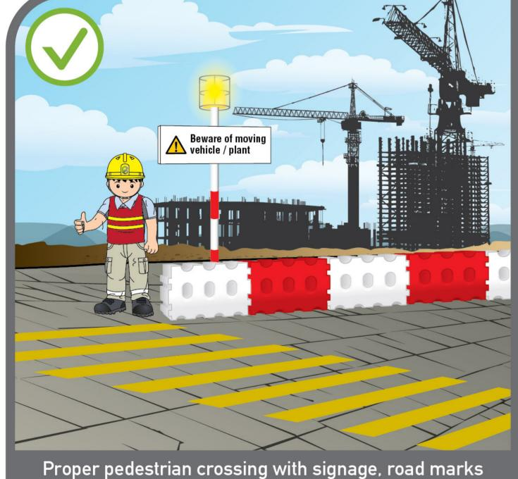
Proper pedestrian crossing with signage, road marks and flash lights on construction sites.
