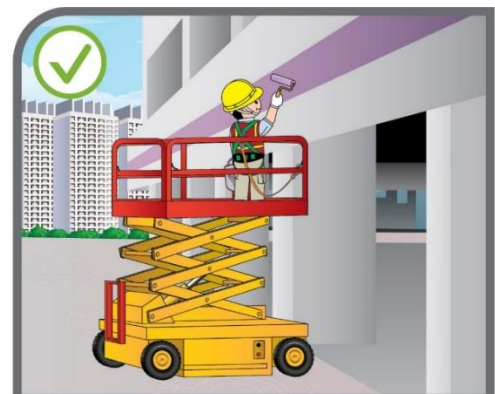
Use suitable working platforms, for example, power-operated elevating working platform or mobile working platform
