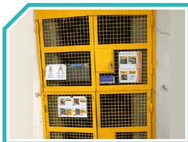
Installation of Four leaf of lift shaft gates as an essential safety measure for lift shaft
