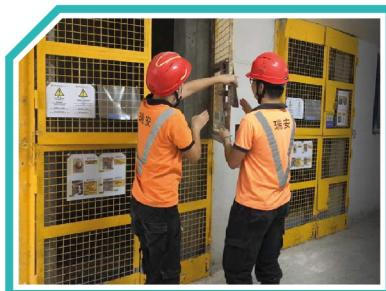
Detection by the NB-IoT sensor and triggering a alert signal to the control office and officer-in-charge for follow-up action when there is unauthorised opening of the gate.
