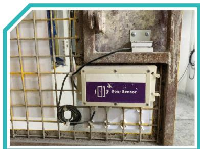
Installation of NB-IoT senor on the inner side of the door
