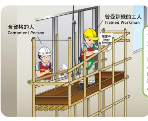
竹棚架的架設/攜建/更改/拆 卸工作須由曾受訓練的工人在 合資格的人直接監督下進行。 Bamboo scaffolds shall be erected. added to, altered or dismantled by trained workmen under the immediate supervision of a competent person.
