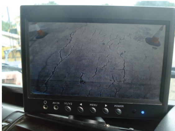
Figure 2 – Typical Image Displayed on Monitor
