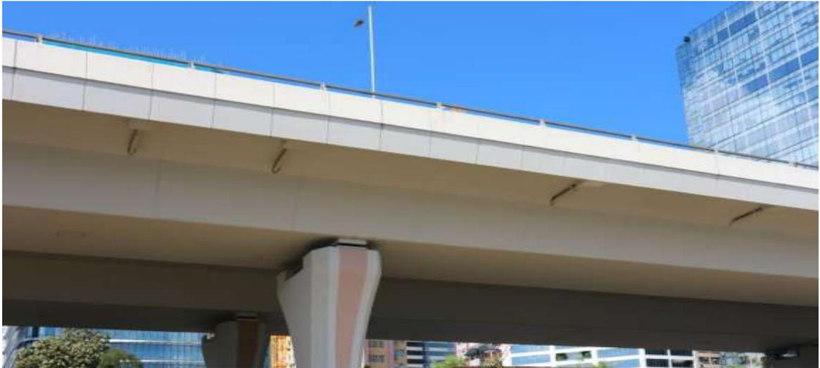
**Figure 1.5 A typical girder bridge**
