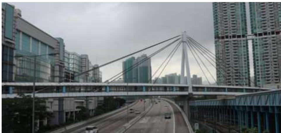
**Figure 1.8 Pedestrian cable-stayed bridge over West Kowloon Highway at Olympic**
