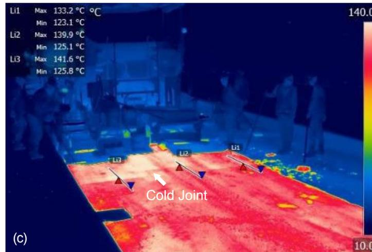
Figure 33(c) Thermal Image of the Asphalt Pavement during Paving
