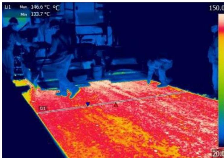
Figure 30 Temperature Monitoring During Paving
