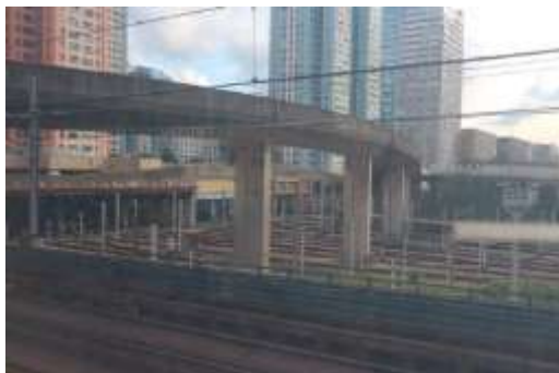
(a) West Kowloon Corridor Span 7/1N-7/27N: M-beam deck, "Y"-shaped pier
