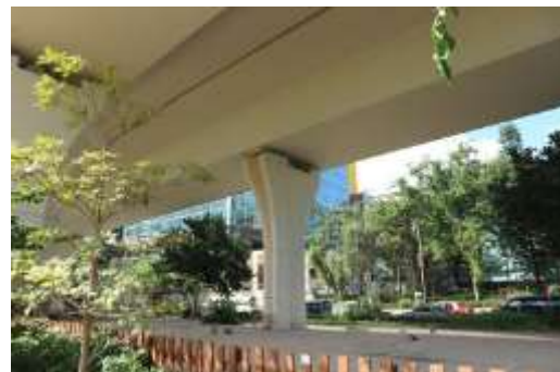
(b) Island Eastern Corridor: U-beam deck, twin-column bent pier
