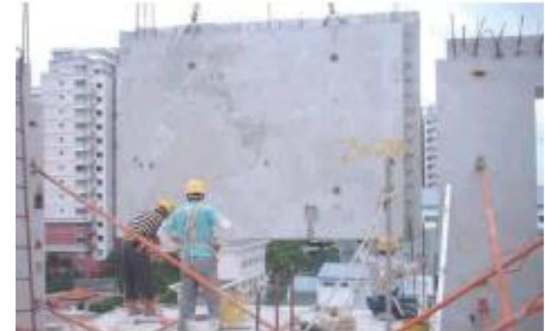
Fig. 6.9 – Lowering of precast wall panel during installation
