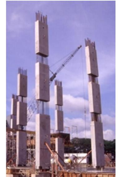
Precast Columns connected with grout filled pipe sleeve
