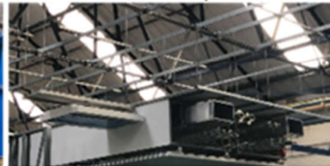
Prefab horizontal module with ceiling board
