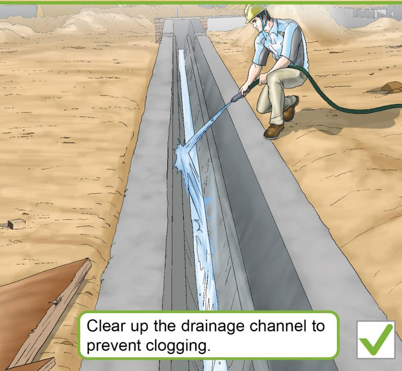
Clear up the drainage channel to prevent clogging.
