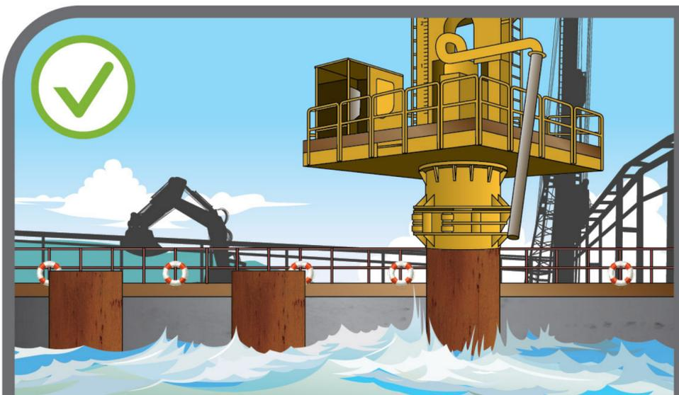
Suitable working platforms, guard-rails and toe-boards shall be provided to machinery used over water.
