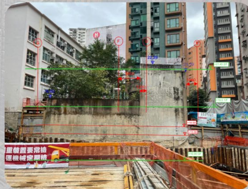
Precast façade panel at external wall facing Brilliant Court to minimize disruption
