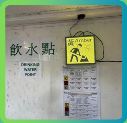
LED Board showing adverse weather warning
