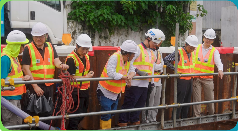
Joint Safety Inspections by CEDD, Consultant and GRJV
