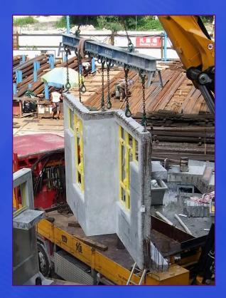
c) Symmetry of layout could also greatly enhance the tower crane capacity as the reach of the crane can be optimized. Sometimes, if the block is very asymmetric, two instead of one tower crane may be required.
