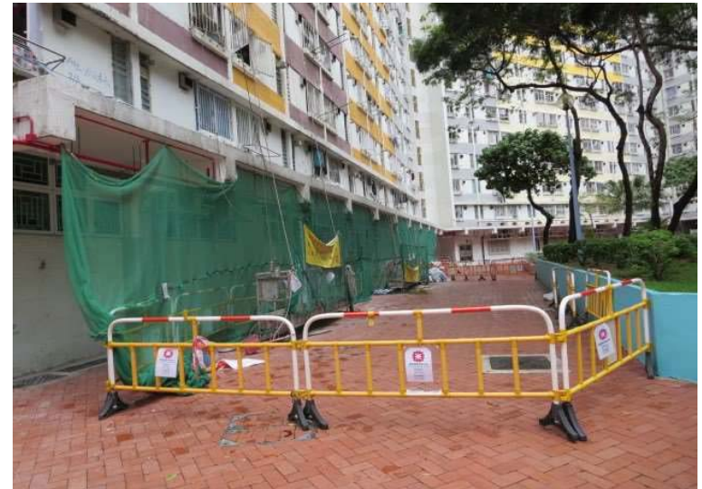
f) Fencing off the works area
