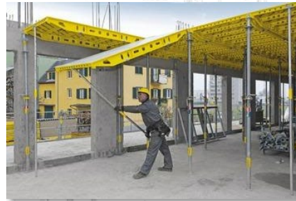
System Formwork
