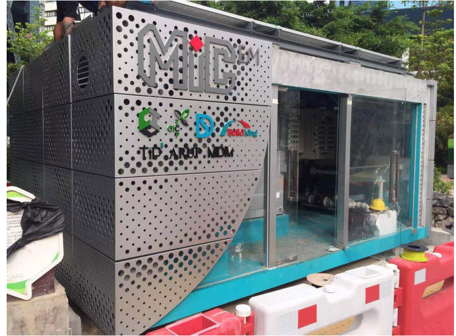
MiC Water Cooling Chiller Plant at CIC Zero Carbon Park
