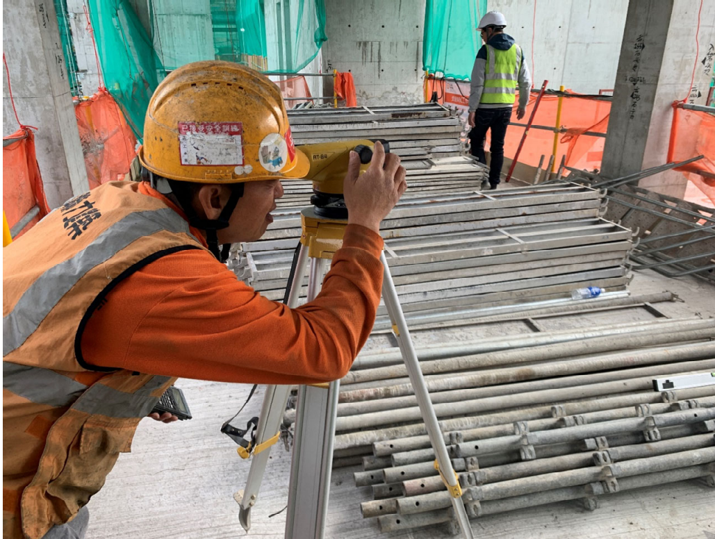
Verification of floor level for module installation
