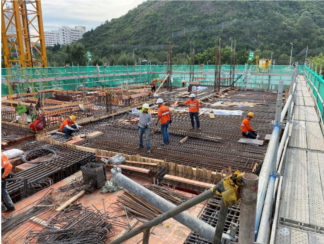
5. Transfer floor construction – Late Oct, 2019
