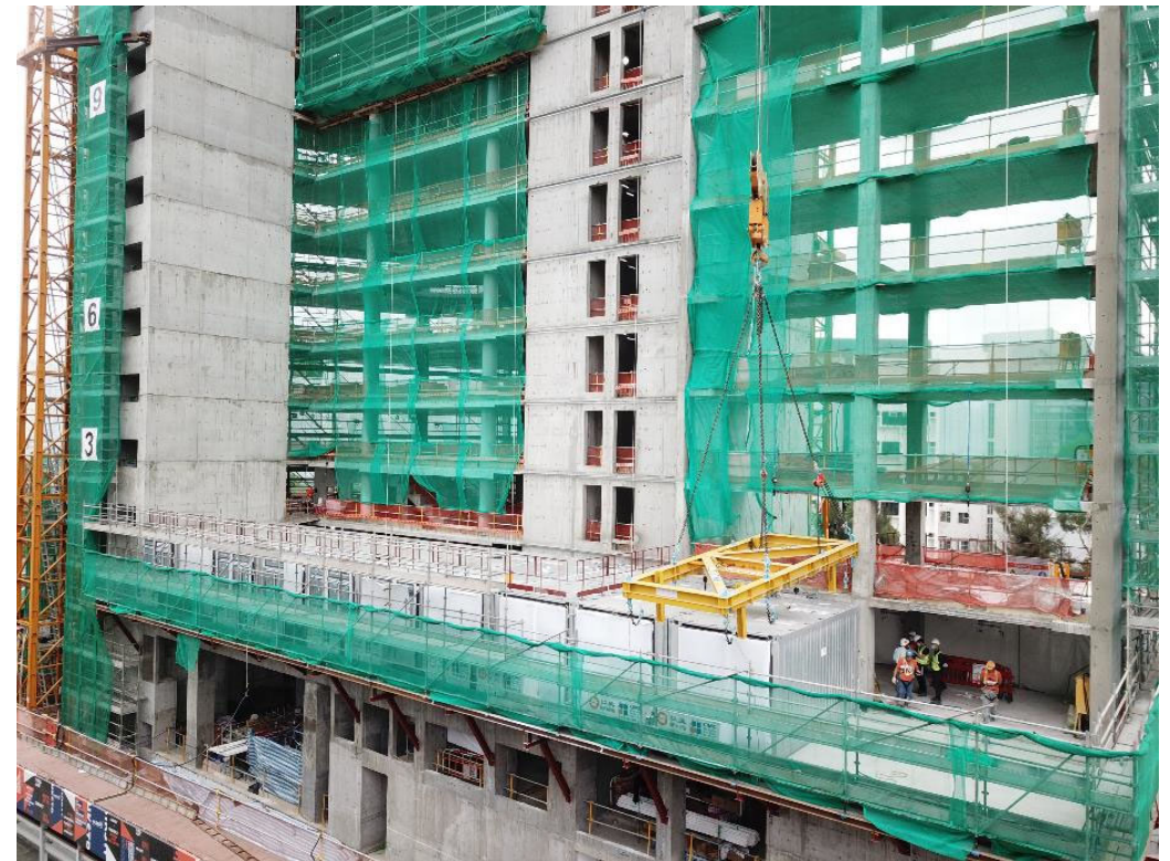
8. Module installation– Late Jan, 2020
