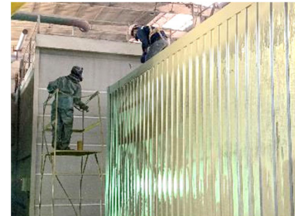
8. Application of anti-corrosion paint at weld joints
