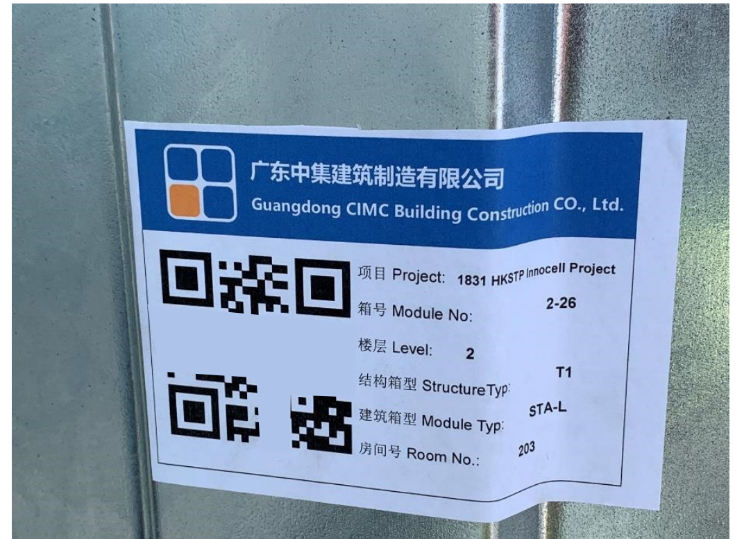
Unique marking for each module
