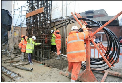
Geothermal Loop and Energy Piles
