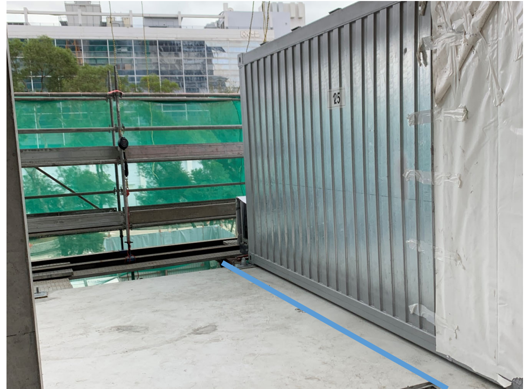
Reference lines for checking of alignment
