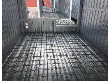
11. Rebar fixing
