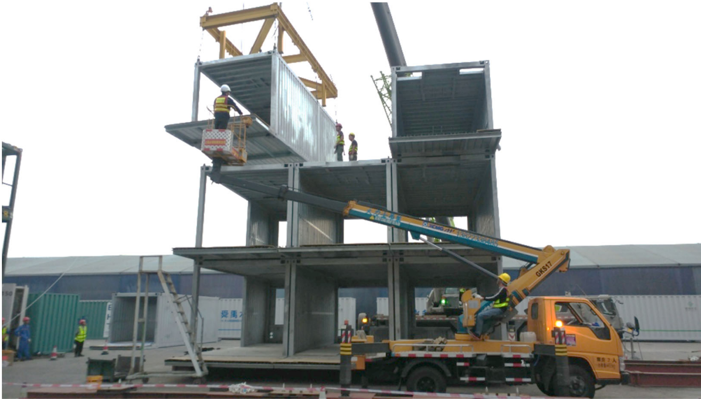
Trial module assembly
