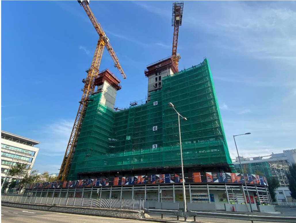
7. Core wall construction – Early Jan, 2020
