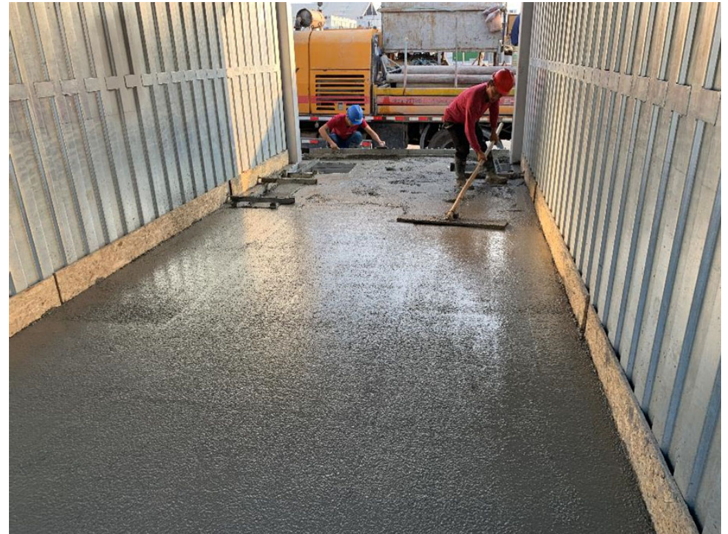
12. Concreting (~0.5 days)
