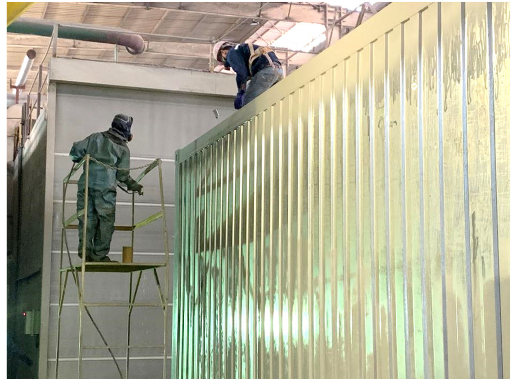
8. Application of anti-corrosion paint at weld joints (~0.5 days)
