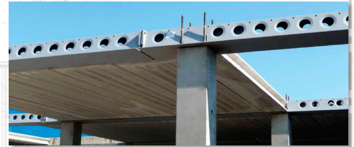
Delta Beam + Hollowcore Precast Pre-stressed Plank
