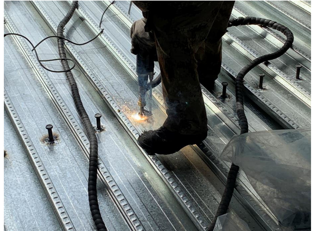
10. Shear studs welding (~0.5 days)
