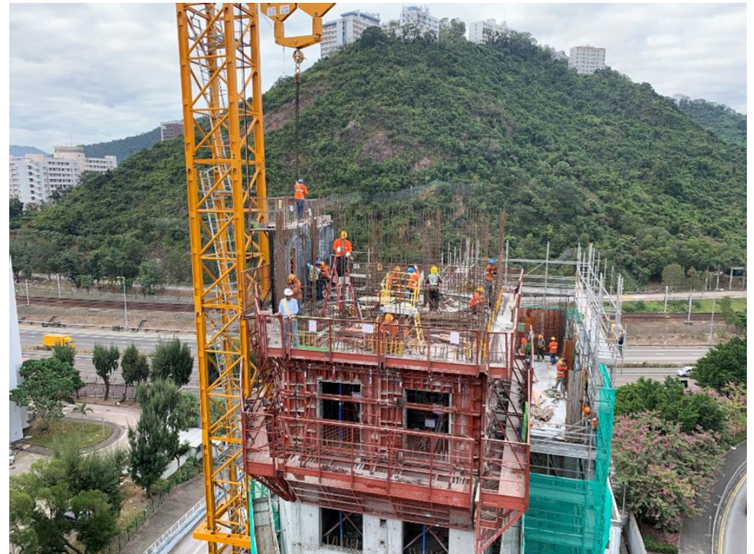
6. Core wall construction – Mid Dec, 2019
