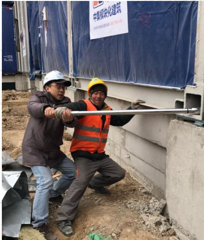
Tighten Preloaded Bolt by Manual Torque Wrench
