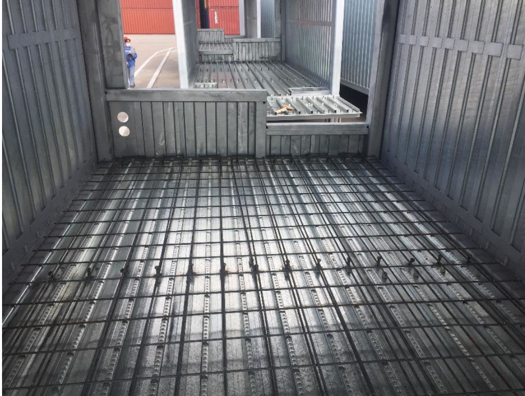
11. Rebar fixing (~0.5 days)
