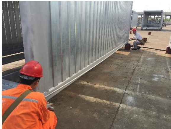
Measurement of module size
