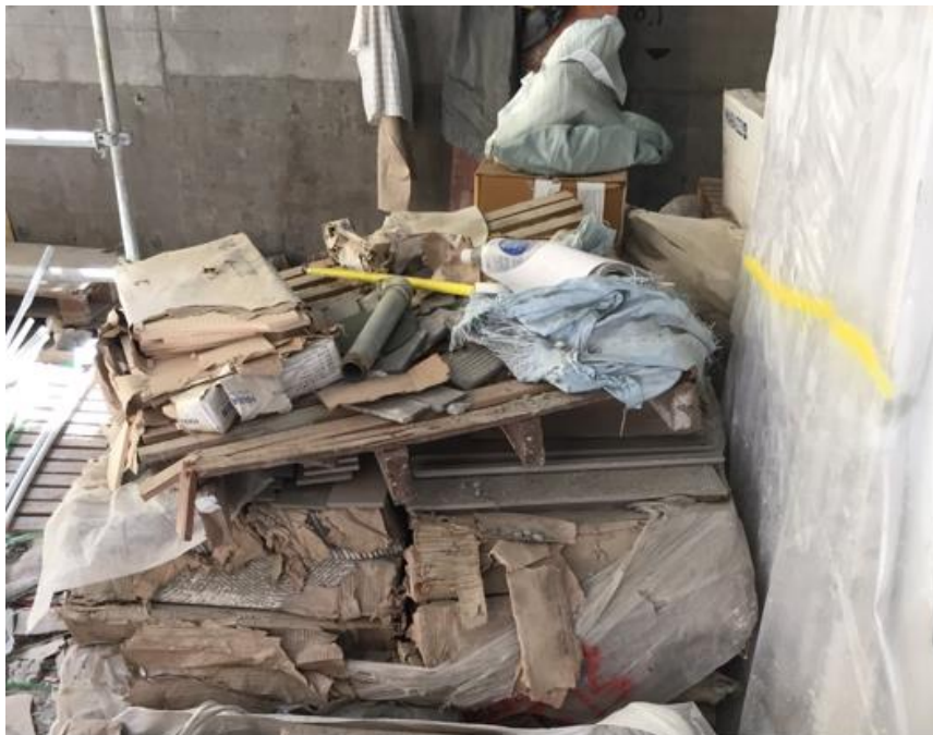
Photo 1 Site visit at Site A
