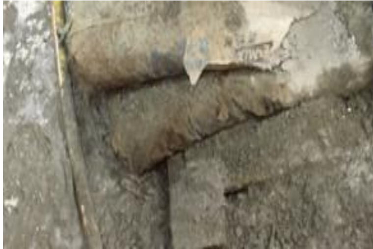
Photo 21: Damaged Bolding Agent due to Water
