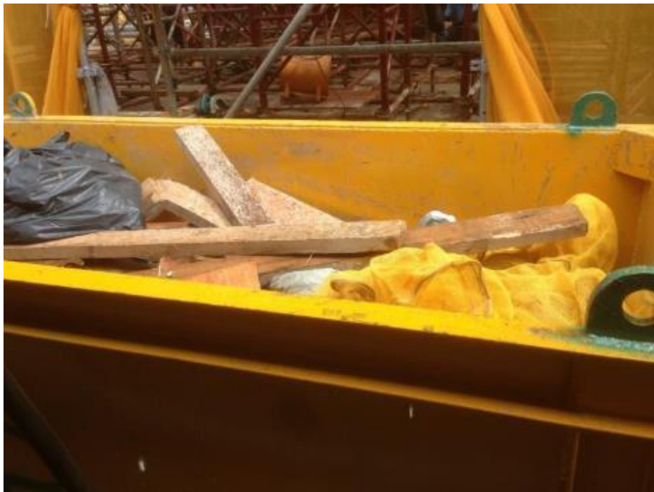
Photo 84: Contents of Construction Waste in Skip B (Mainly Consisting of Nylon Net, Timber etc.)
