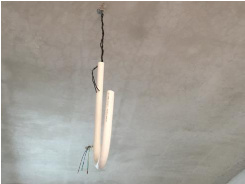
Photo 2: Electrical Connection Setting (2)
