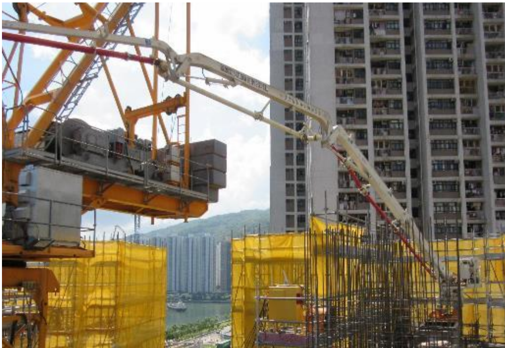
Photo 46: Concreting by Pumping
