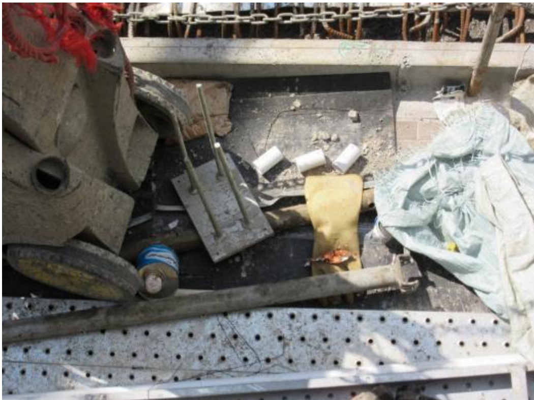
Photo 52: Construction Wastes Noted Near to Concreting Area
