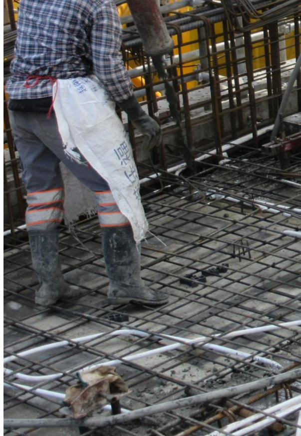
Photo 47: Concreting – in Progress
