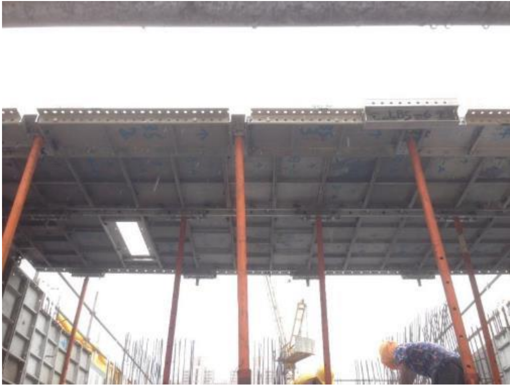
Photo 76: Installation of Aluminium Formwork (3)
