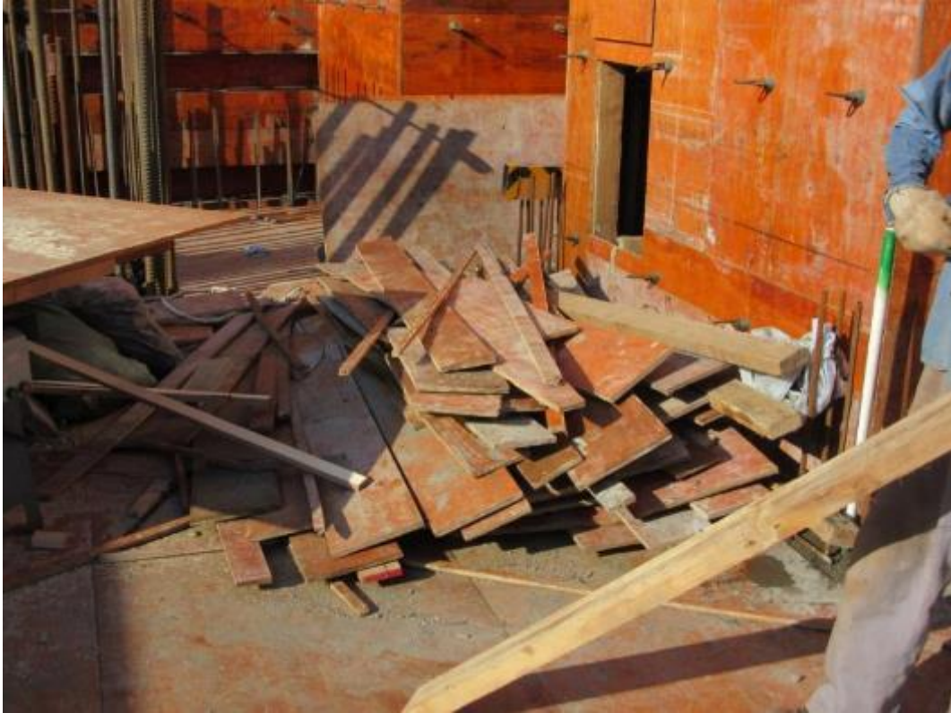
Photo 71: Scraped Timber to be Reused on Site
