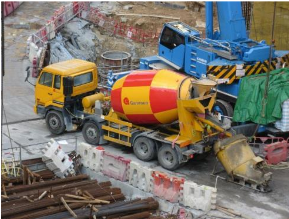
Photo 50: Concreting by “Crane + skip”
