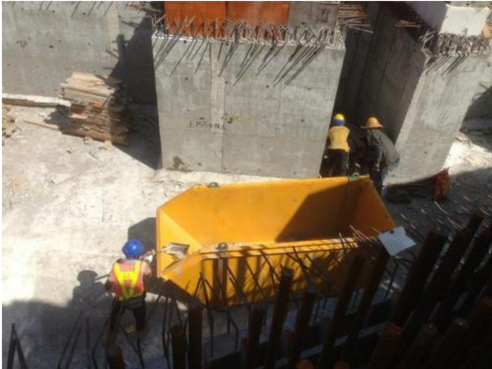
Photo 91: Large Skip for Collecting Waste at Ground Level
