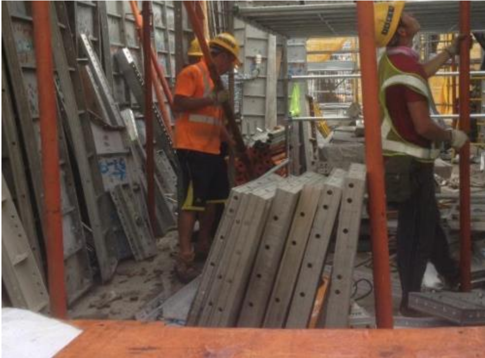
Photo 74: Installing of Aluminium Formwork (1)
