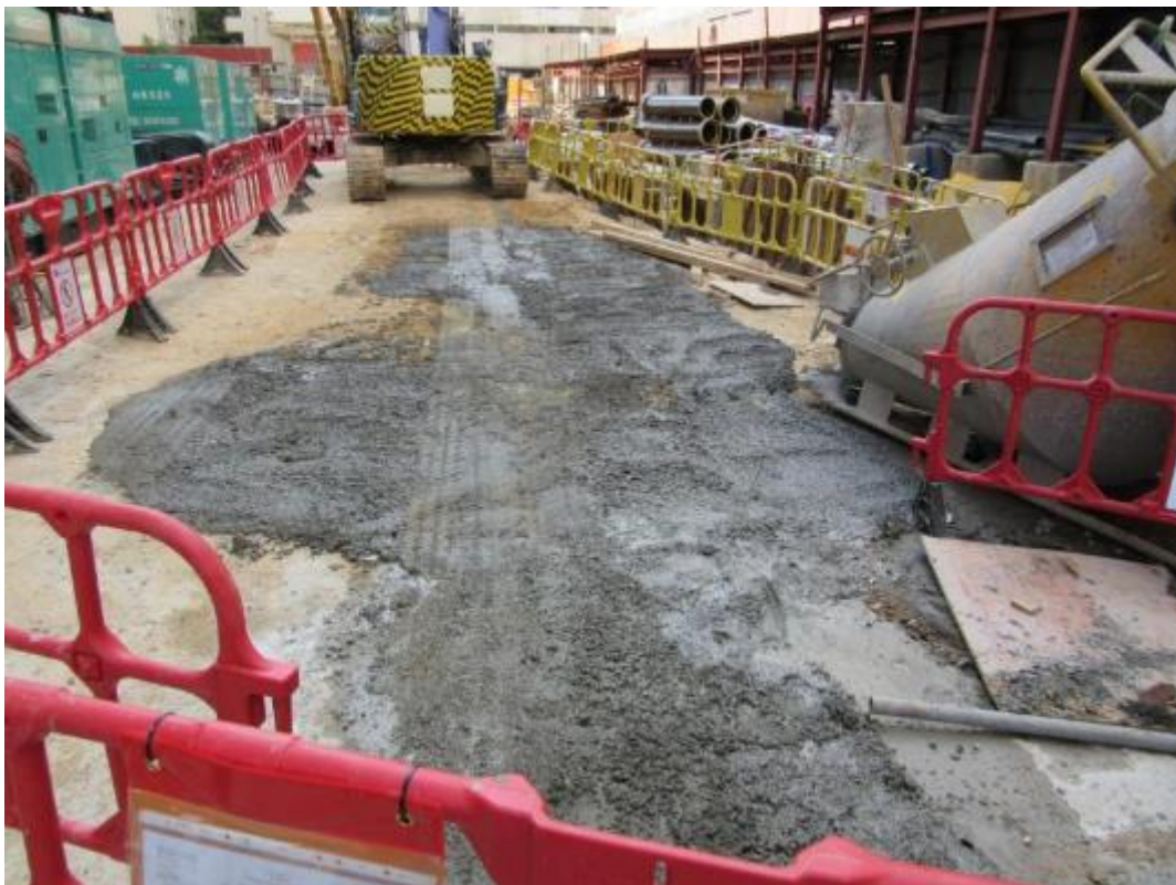
Photo 68: Surplus Concrete for Paving Temporary Access
