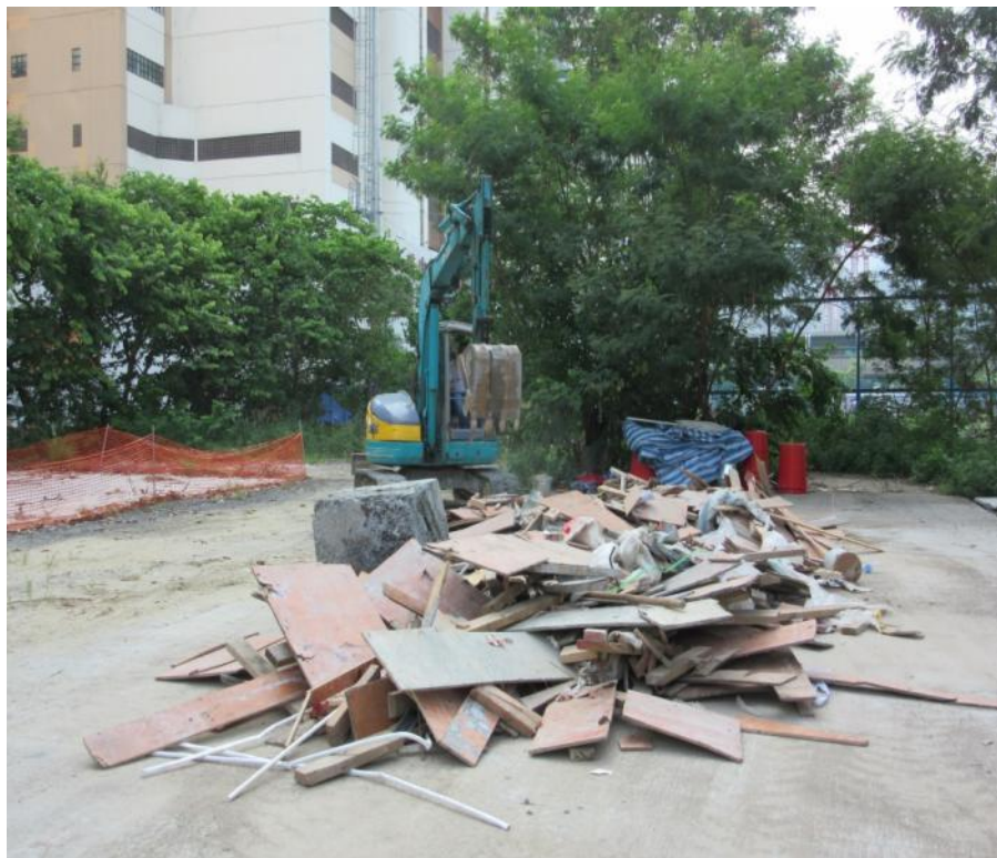
Photo A4: Debris from Site B (II)
