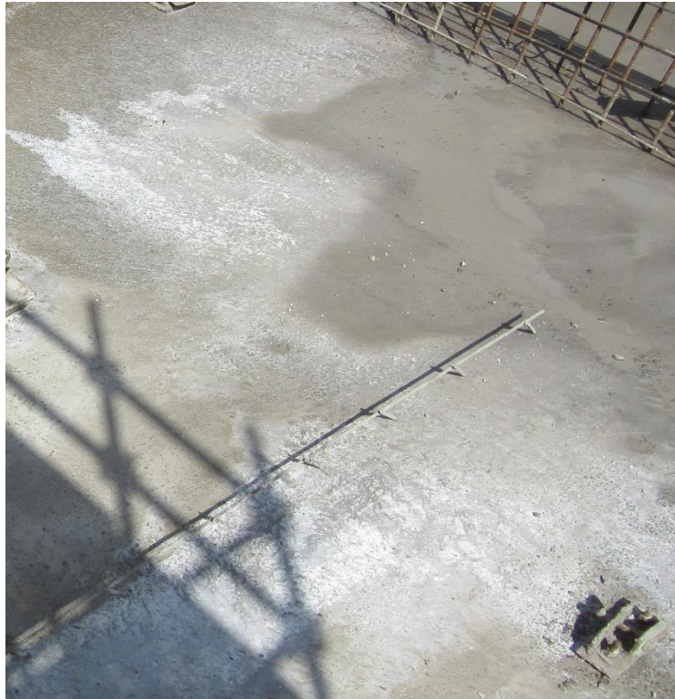
Photo 49: Completion of Concreting
