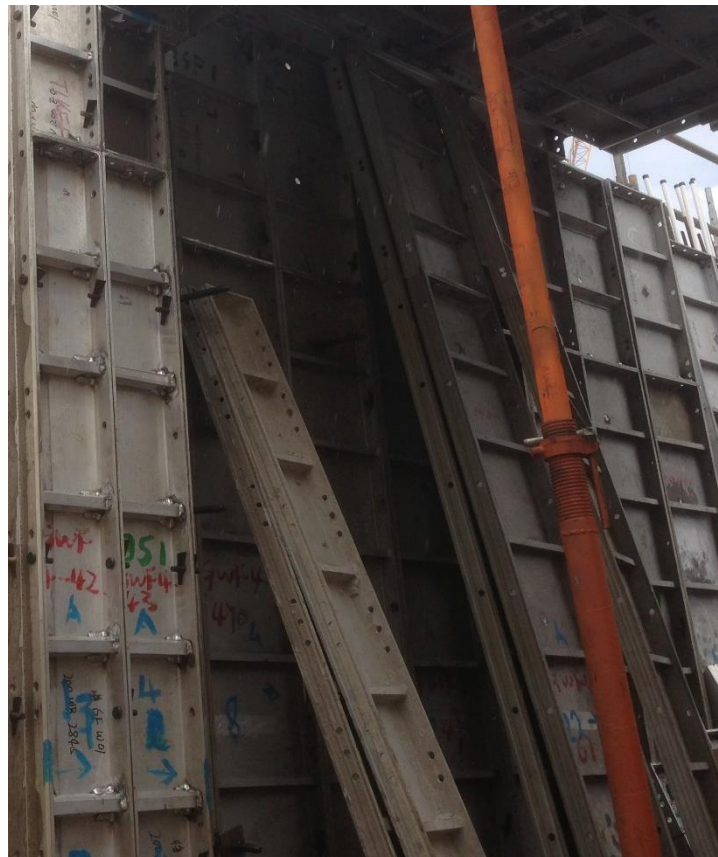
Photo 75: Installing of Aluminium Formwork (2)
