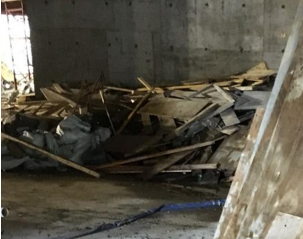
Photo 3 Site visit at Site C
