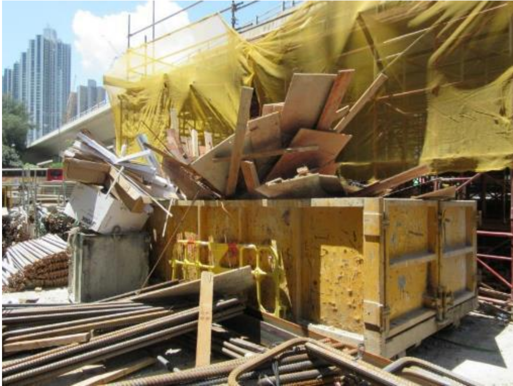
Photo 65: Storing Construction Waste in Skip B
