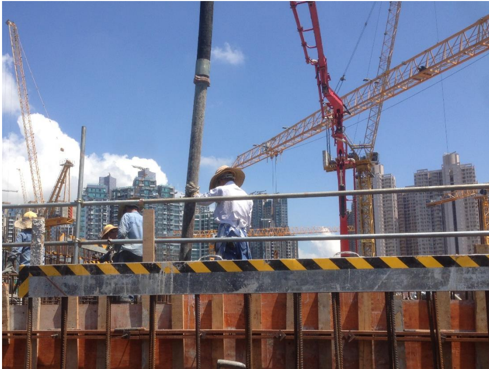
Photo 79: Concreting by Pumping
