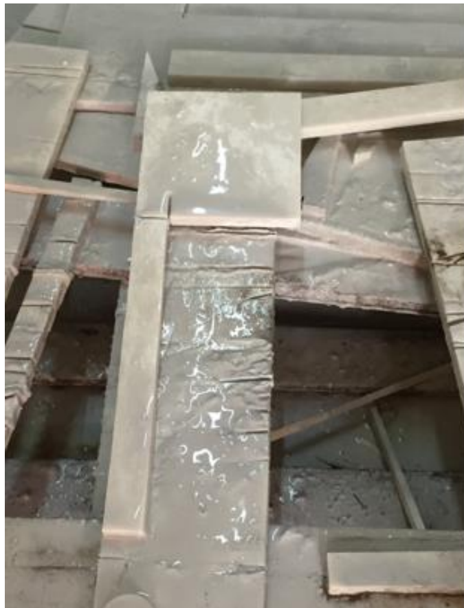
Photo 16: Ends after Tile Cutting
