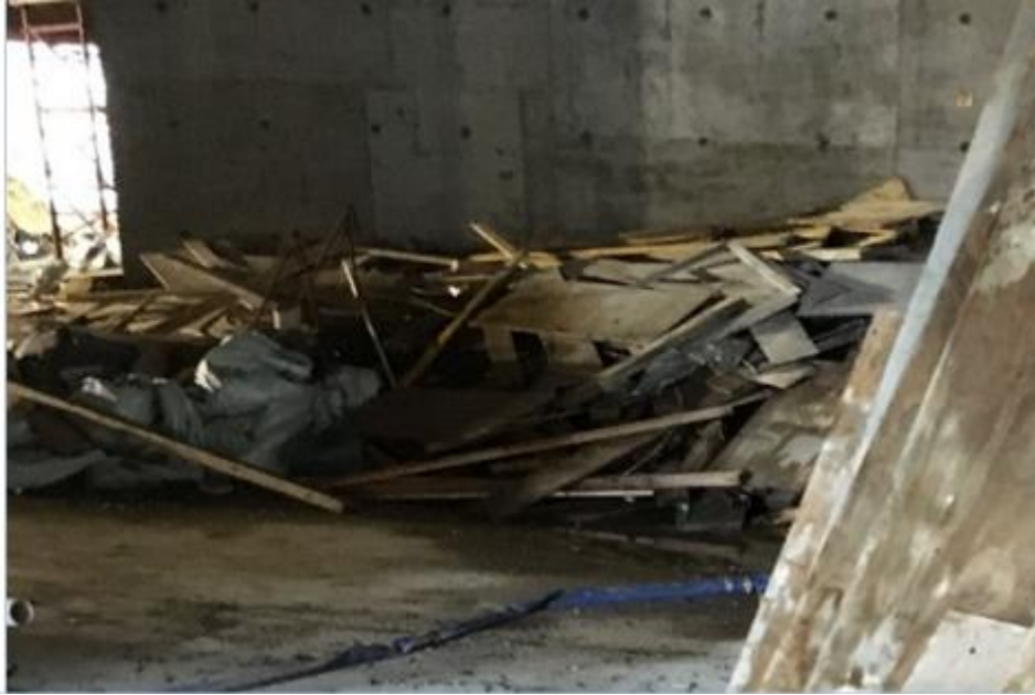
Photo 81: Timber Waste after Removal of Timber Formwork (2)
