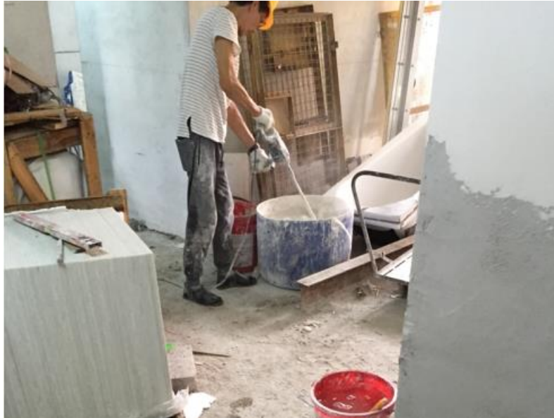
Photo 9: Application of Sealing Primer
