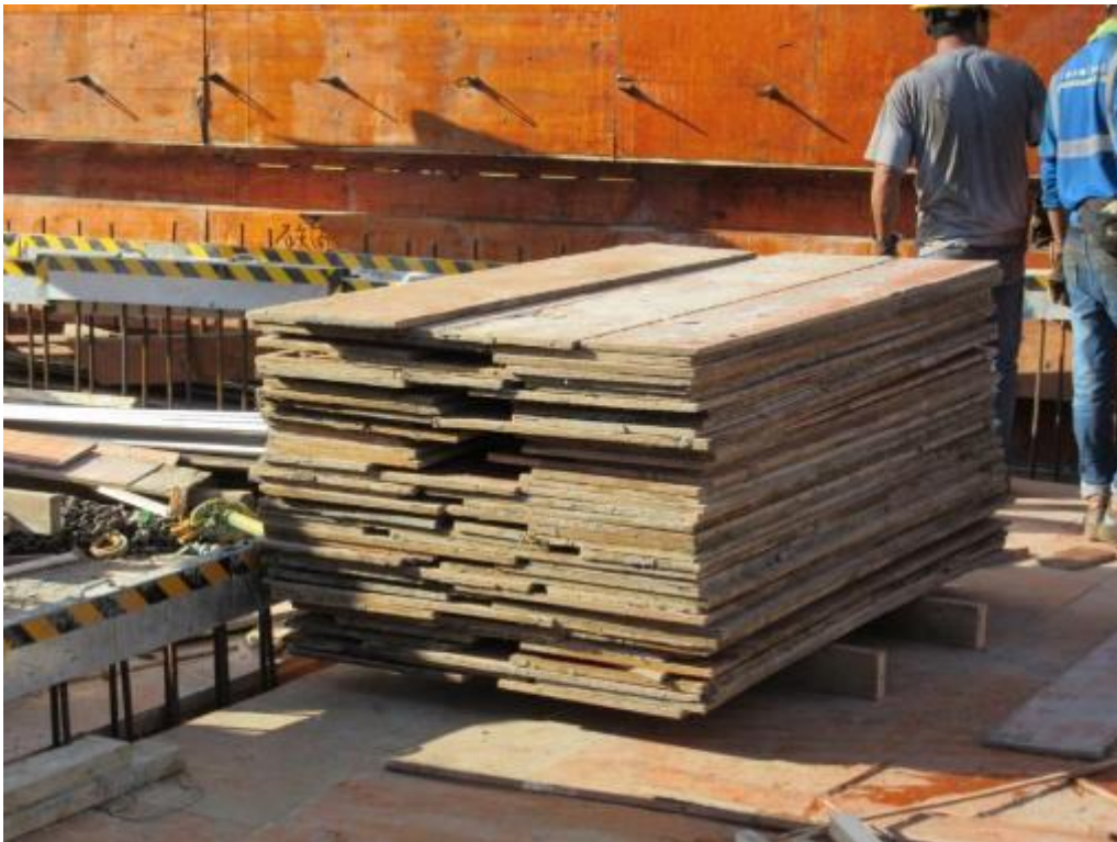
Photo 62: Temporary Storage for Timber
