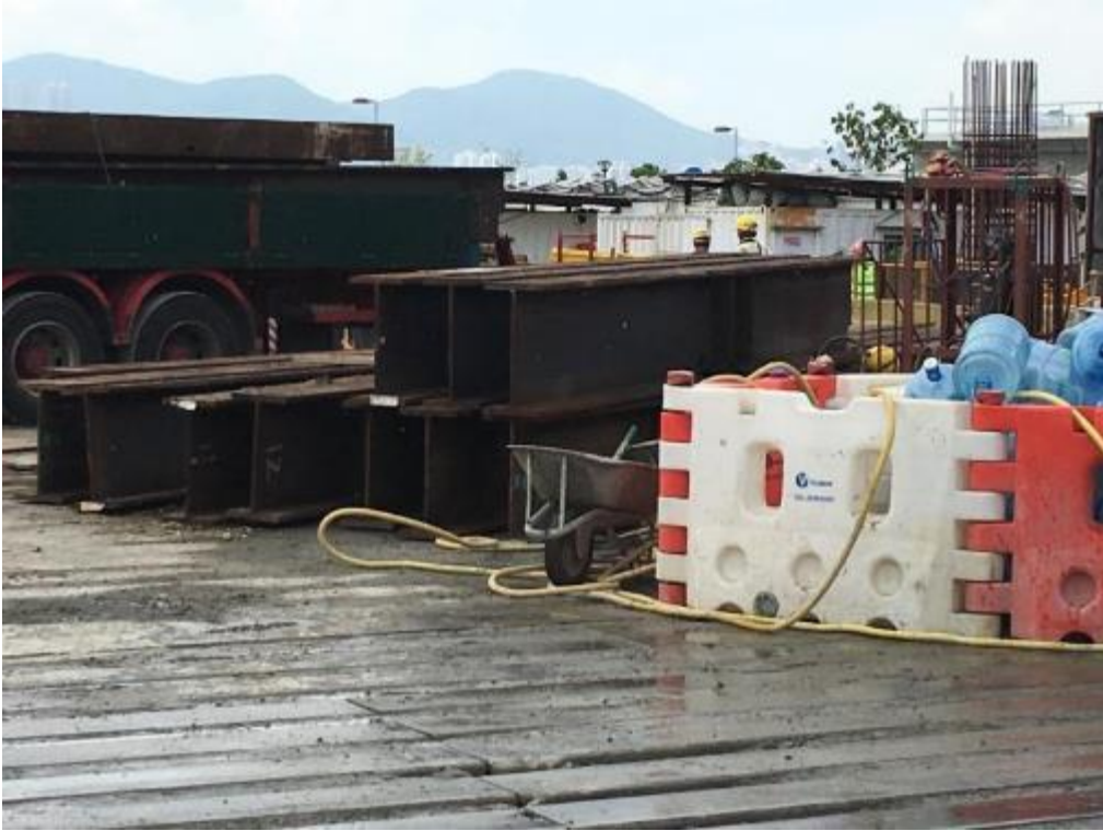
Photo 97: Ends of Steel Beams for Recycling
