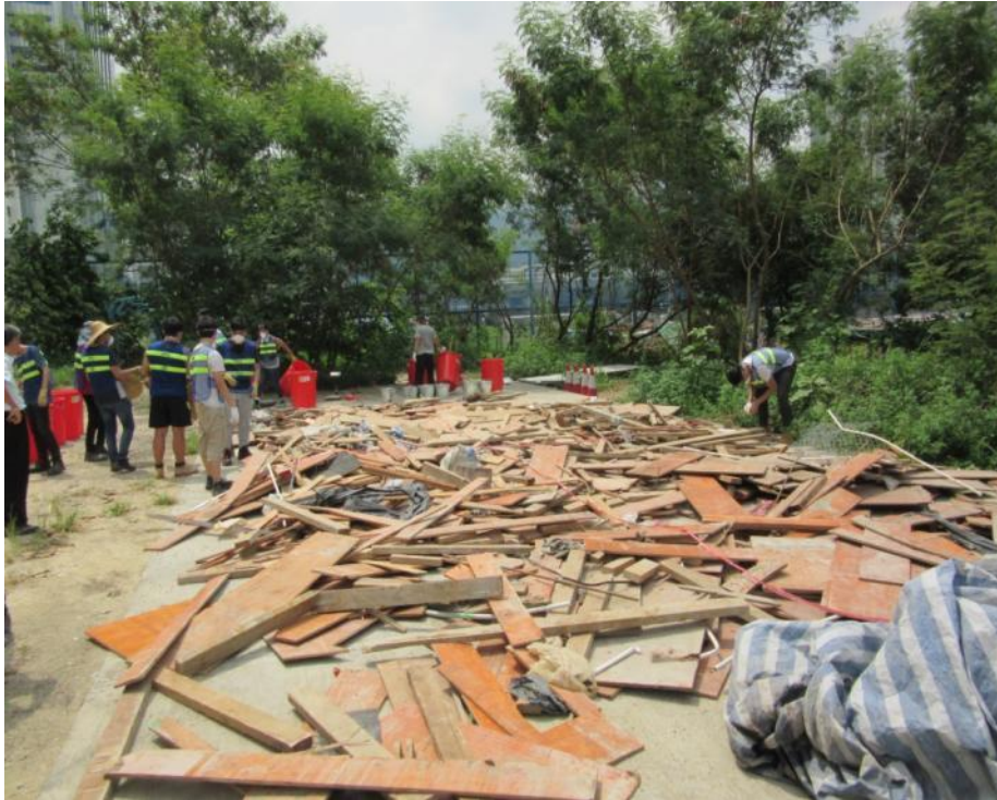
Photo A3: Debris from Site B (I)
