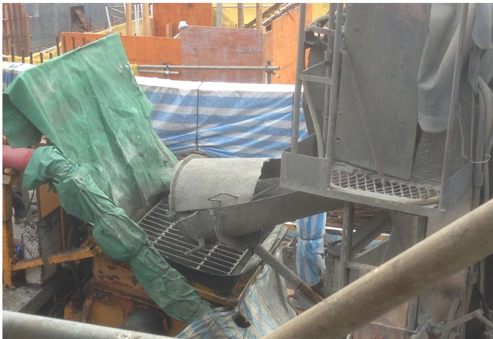
Photo 77: Pouring Concrete to the Pumping Machine
