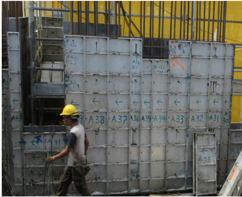
Photo 45: Aluminium System Formwork (2)
