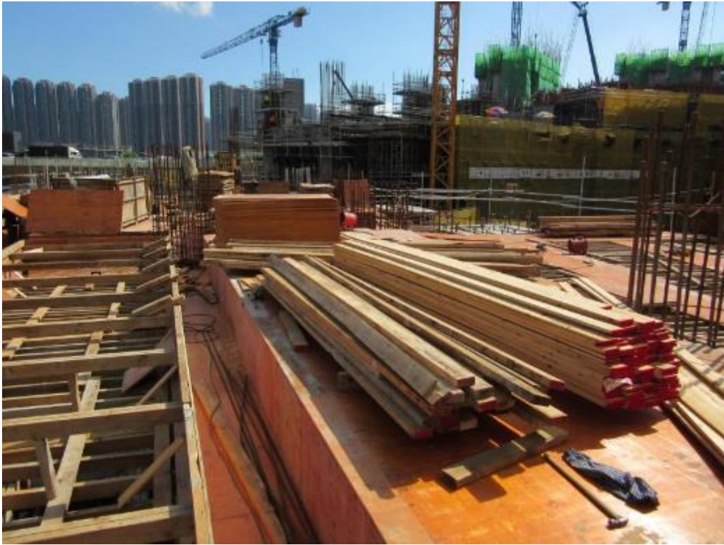
Photo 39: Timber Formwork for Decking of Low-Rise Buildings
