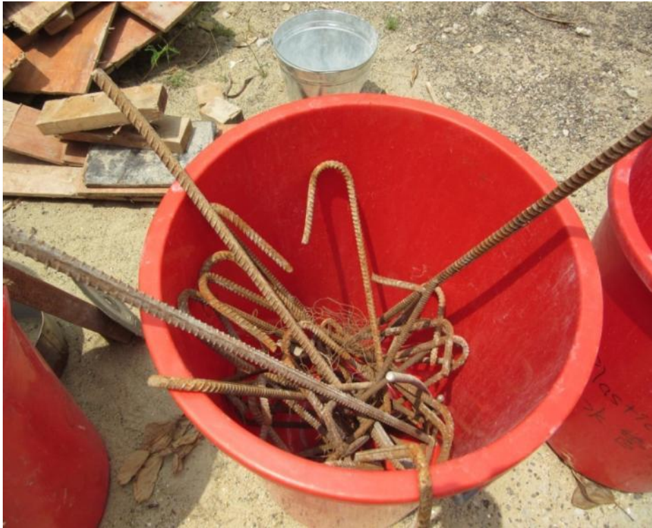
Photo A27: Some Other Construction Waste from Site B (I)
