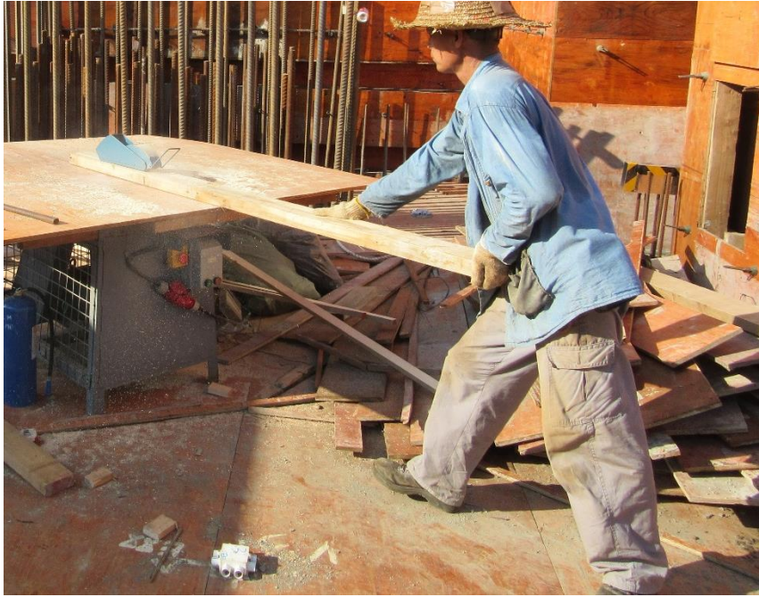
Photo 43: Cutting Timber on Site
