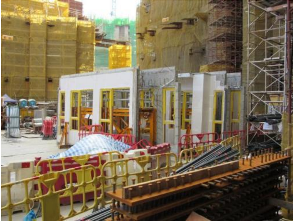
Photo 63: Use of Precast Units
