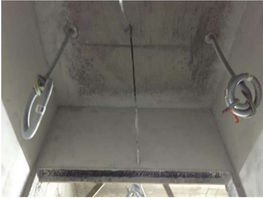
Photo 1: Electrical Connection Setting (1)
