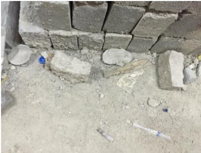
Photo 14: Broken Bricks at a Brickwork Working Area
