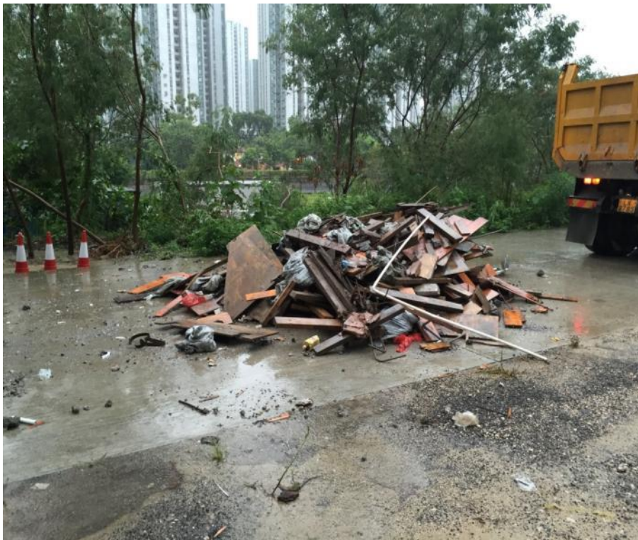
Photo A6: Debris from Site C (II)
