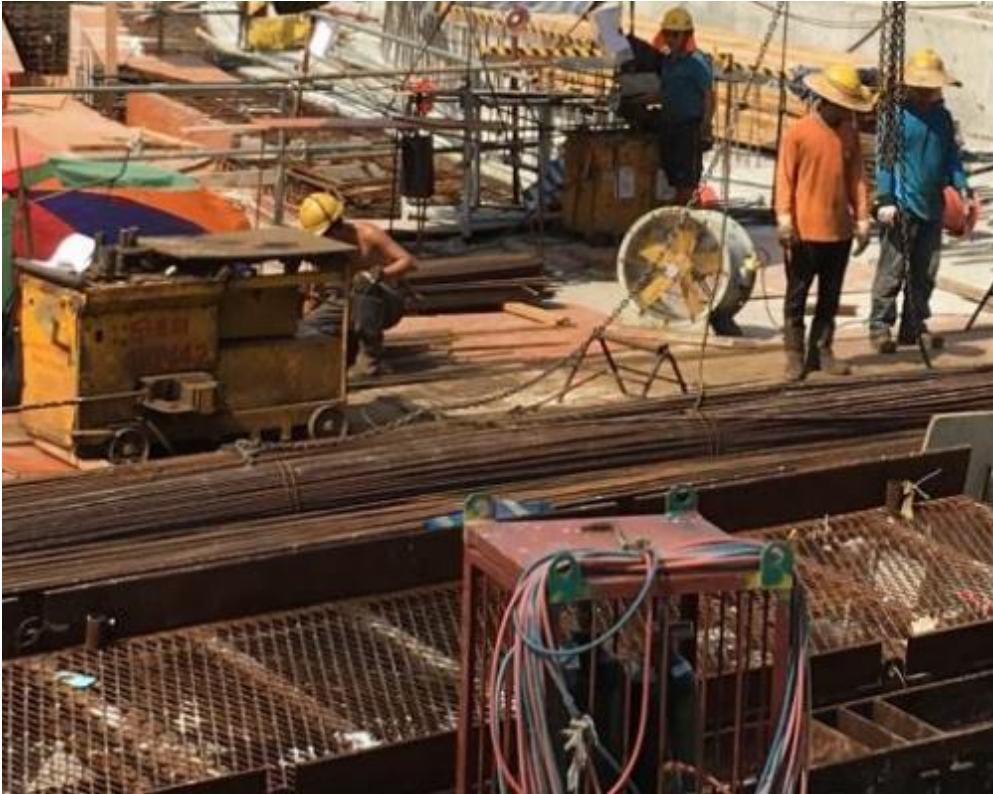
Photo 72: Preparation of Reinforcement Bars
