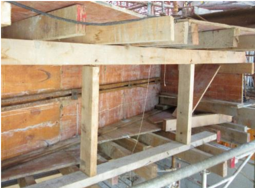
Photo 40: Timber Formwork for Beam of Low-Rise Buildings (1)
