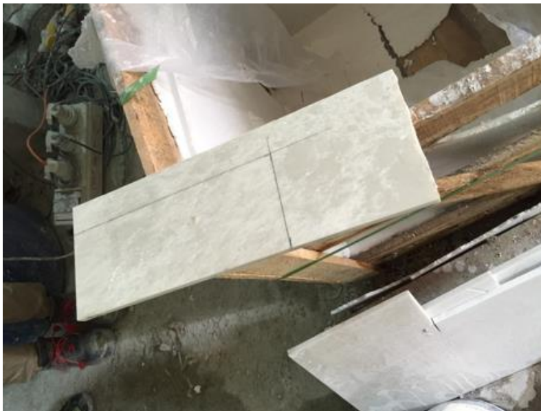
Photo 10: Planning/Measurement before Tile Cutting
