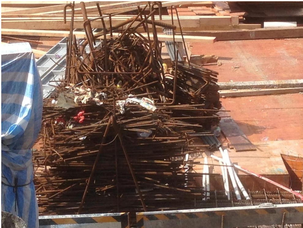
Photo 96: Reinforcement Scraps Sorted for Recycling (2)
