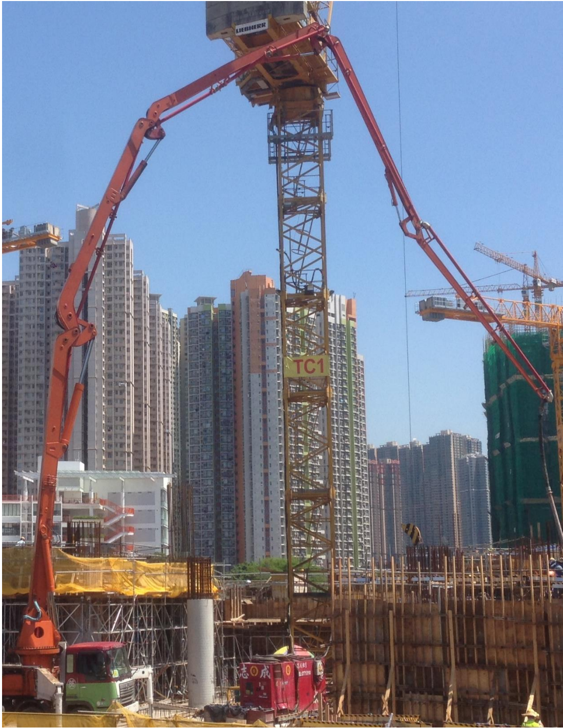
Photo 78: Pipe System of Concrete Pumping Machine
