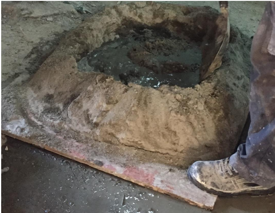
Photo 8: Mixing Materials for Screeding
