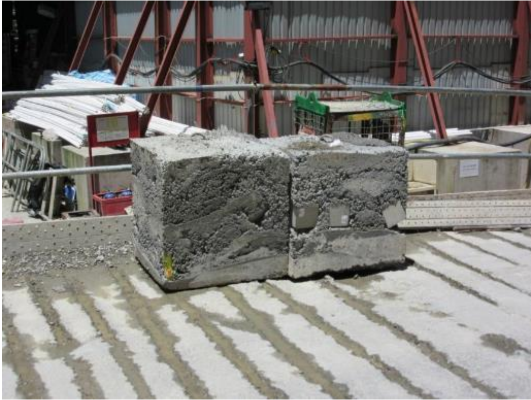
Photo 69: Concrete blocks made of Surplus Material for Temporary Usage
