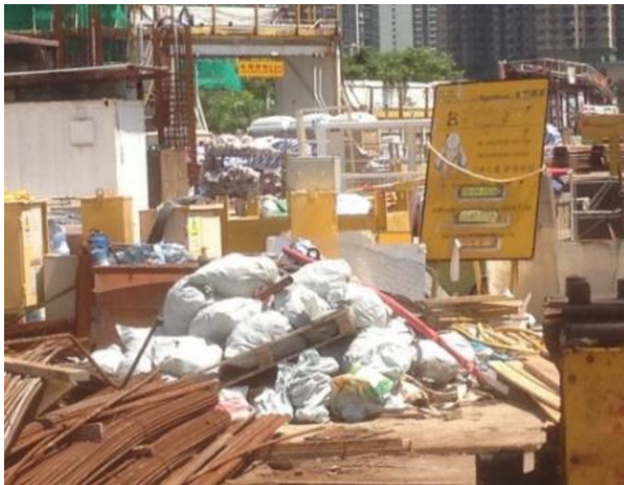
Photo 86: Contents at a Temporary Dumping Location (Mainly Consisting of Timber Pallet, Cable, nylon bags and Steel Scraps etc.)
