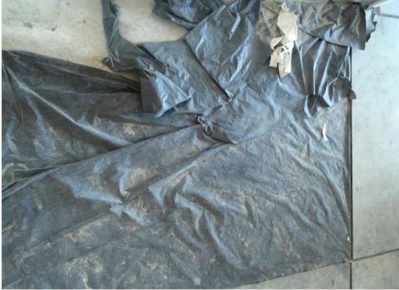
Photo 13: Protection to New Tiled Wall
