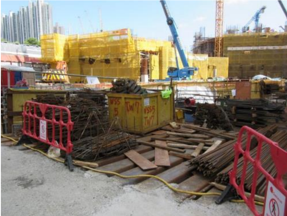
Photo 61: Temporary Storage for Reinforcement Bars
