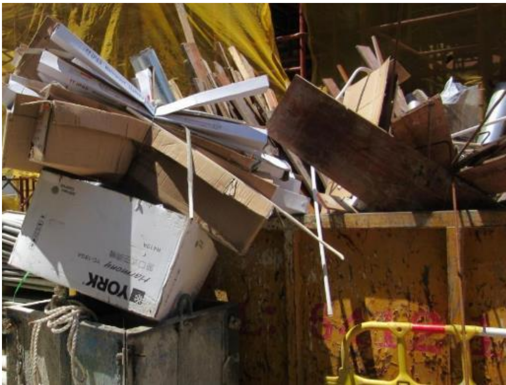
Photo 56: Contents of Construction Waste in Skip B
