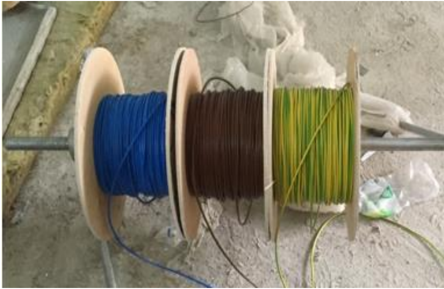
Photo 3: Wires for Electrical System
