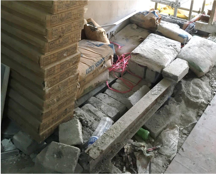
Photo 7: Materials Ready for Brickwork and Tiling
