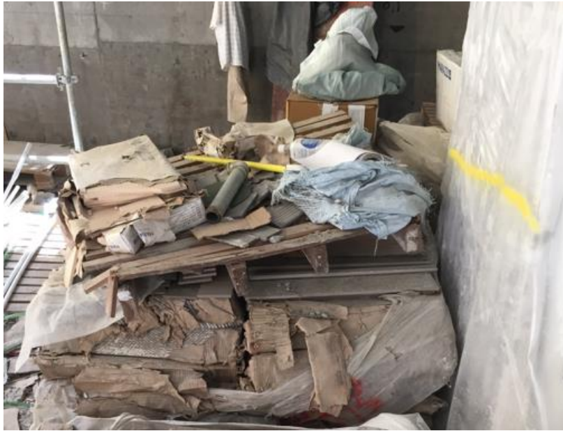
Photo 17: Construction Wastes Noted in a Working Area (1)
