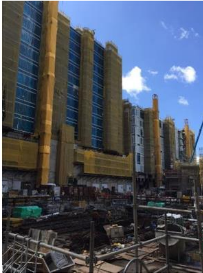
Figure 1 General View of Site A
