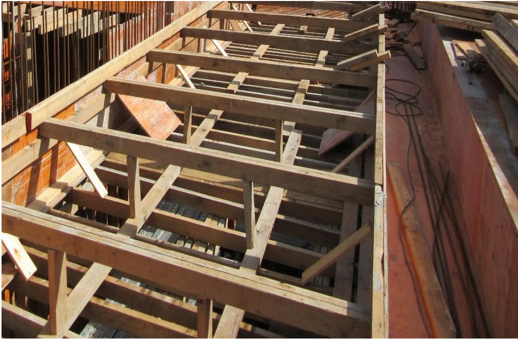
Photo 41: Timber Formwork for Beam of Low-Rise Buildings (2)
