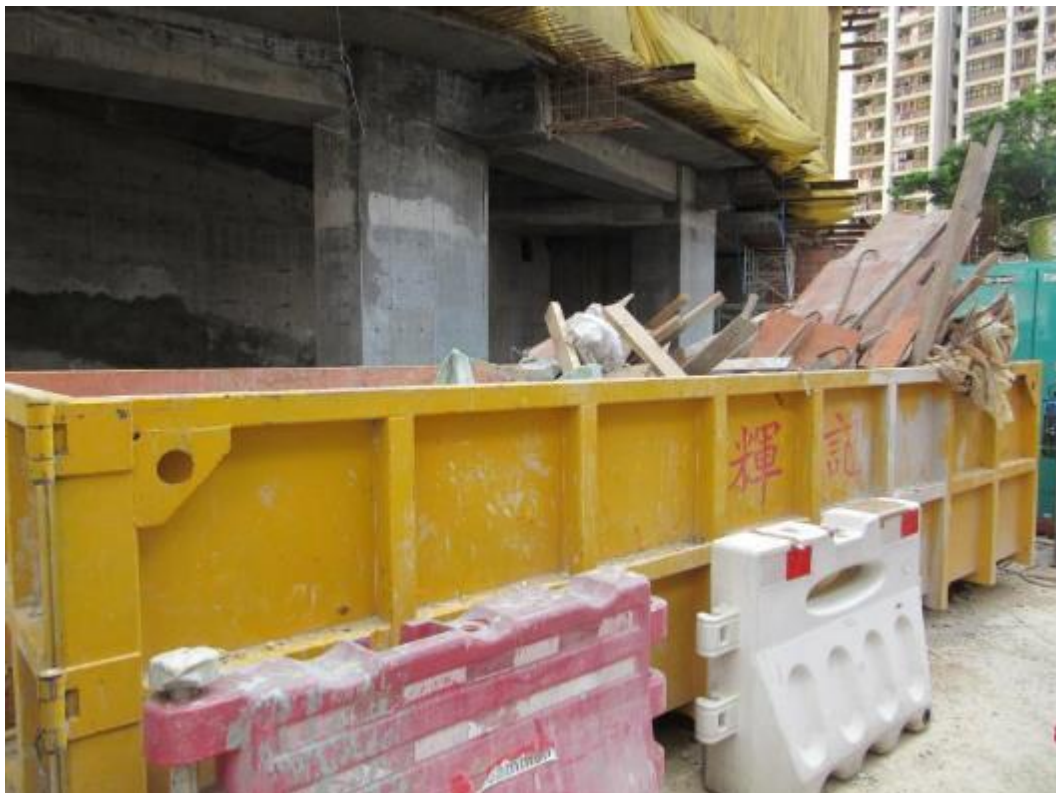
Photo 64: Storing Construction Waste in Skip A
