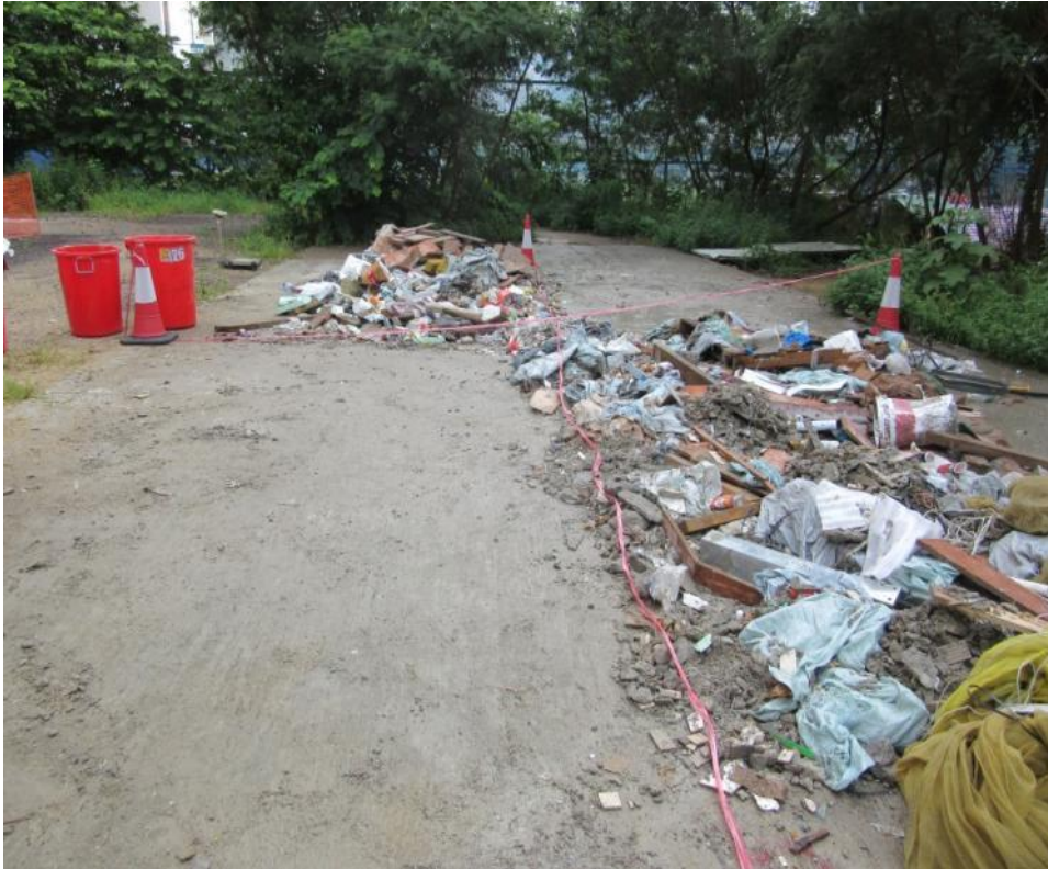
Photo A15: Completion of Sorting (I)
