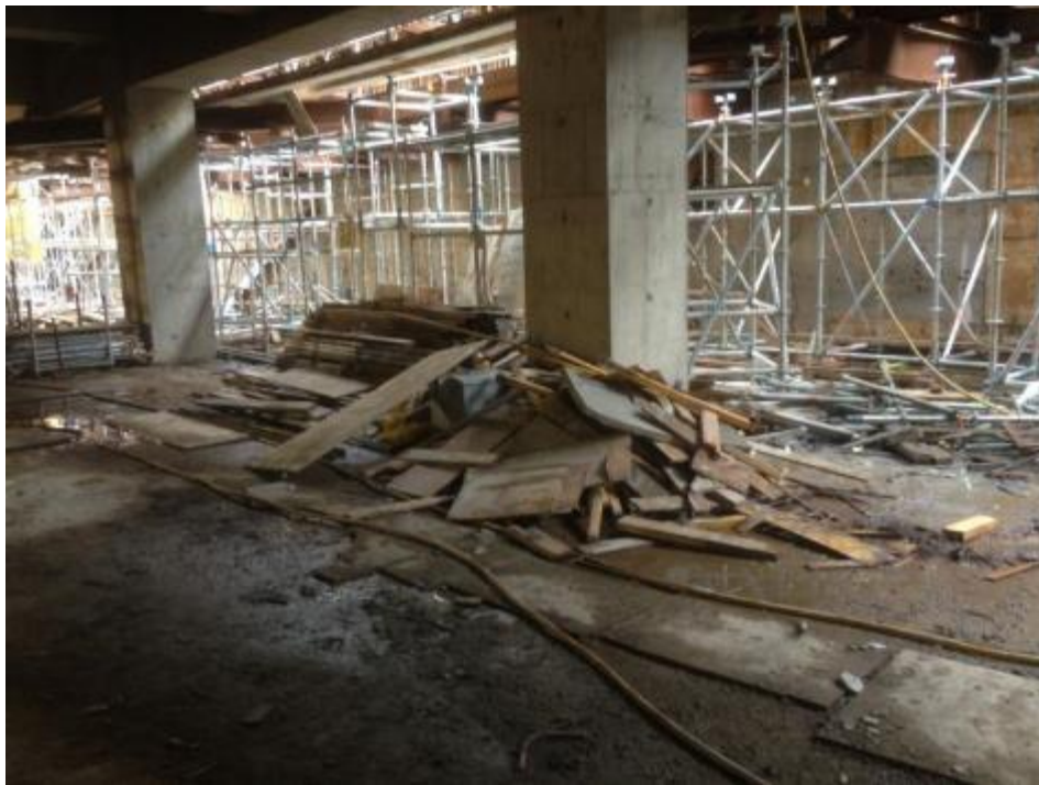
Photo 80: Timber Waste after Removal of Timber Formwork (1)
