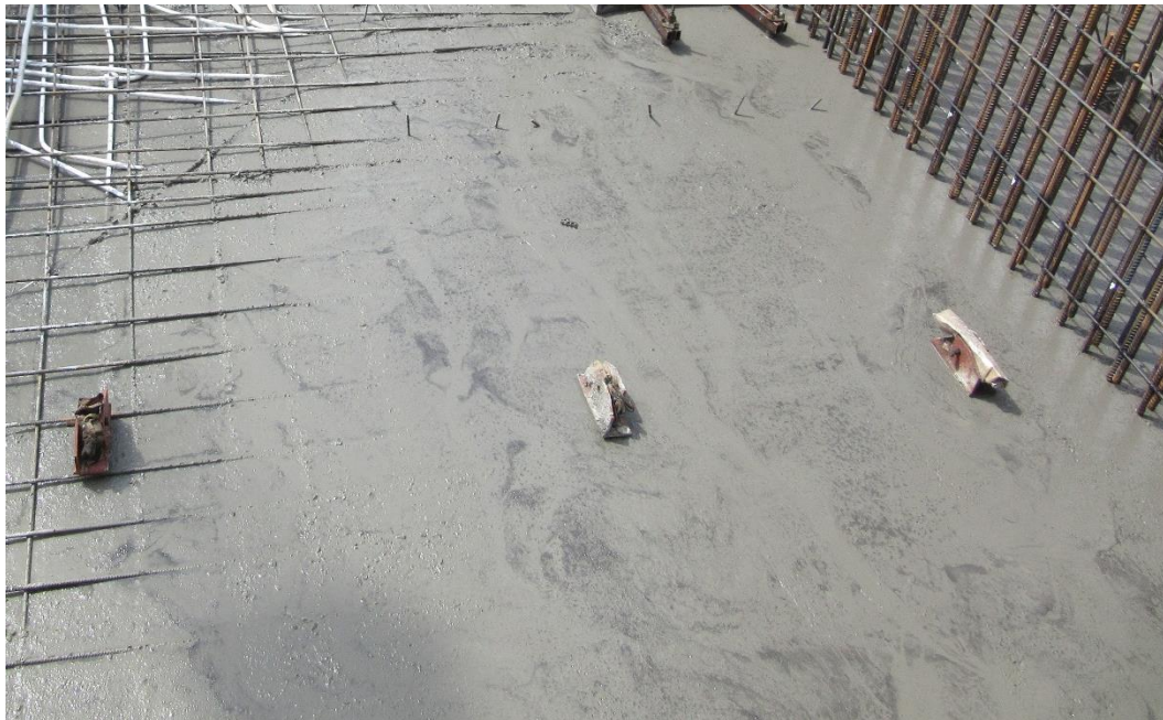
Photo 48: Concreting – Half of the Floor Completed
