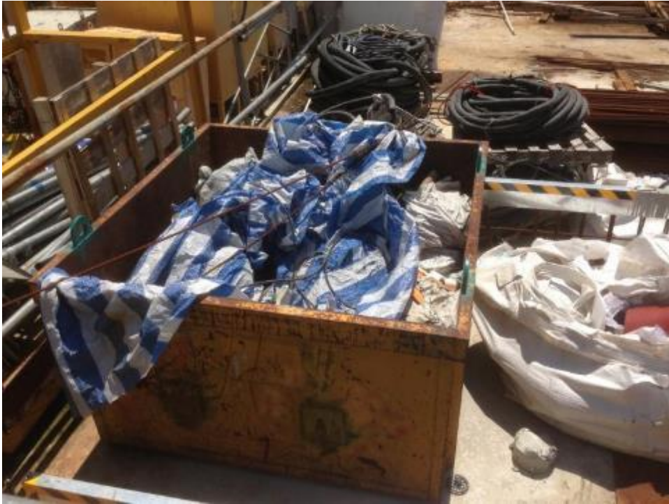
Photo 83: Contents of Construction Waste in Skip A (Mainly Consisting of Nylon Canvas, Steel Bar & Cable etc.)
