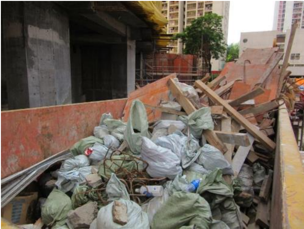
Photo 55: Contents of Construction Waste in Skip A
