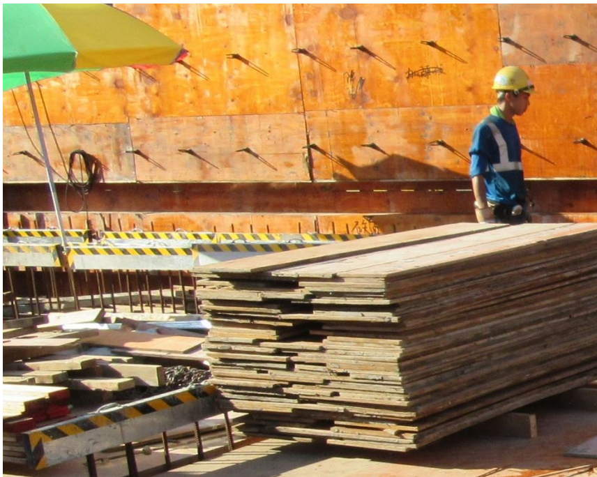
Photo 42: Preparation Area of Timber Formwork
