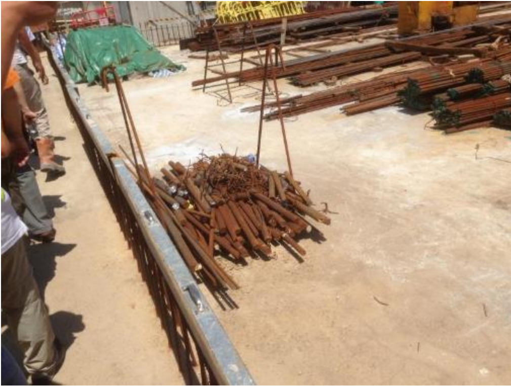
Photo 95: Reinforcement Scraps Sorted for Recycling (1)
