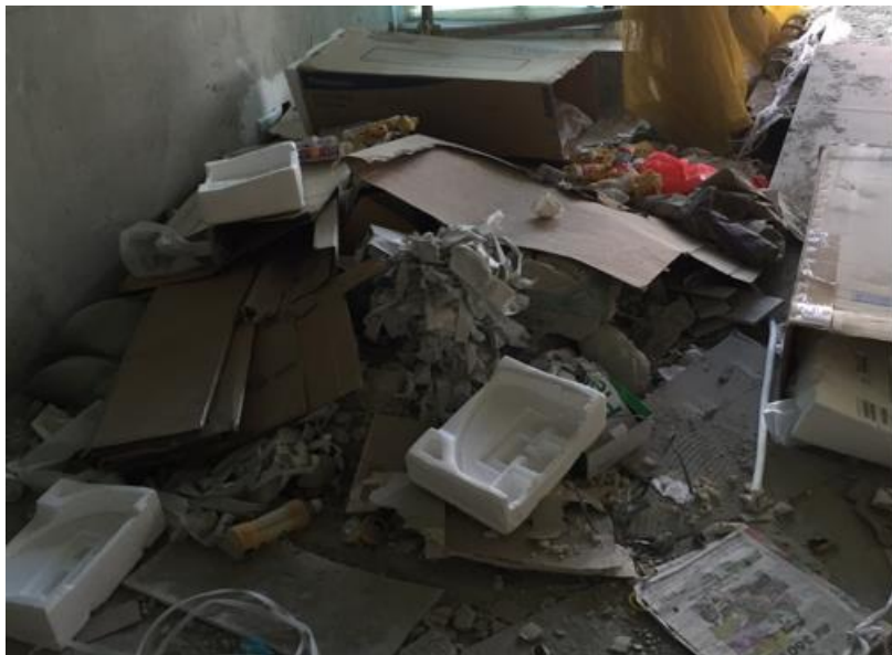
Photo 18: Construction Wastes Noted in a Working area (2)
