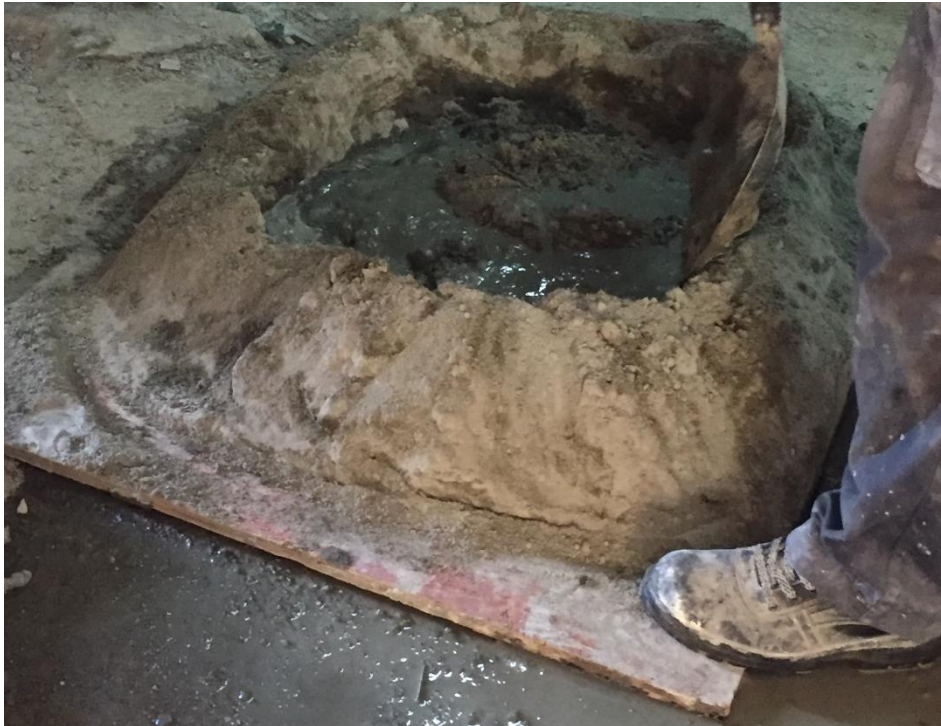
Photo 8: Mixing Materials for Screeding
