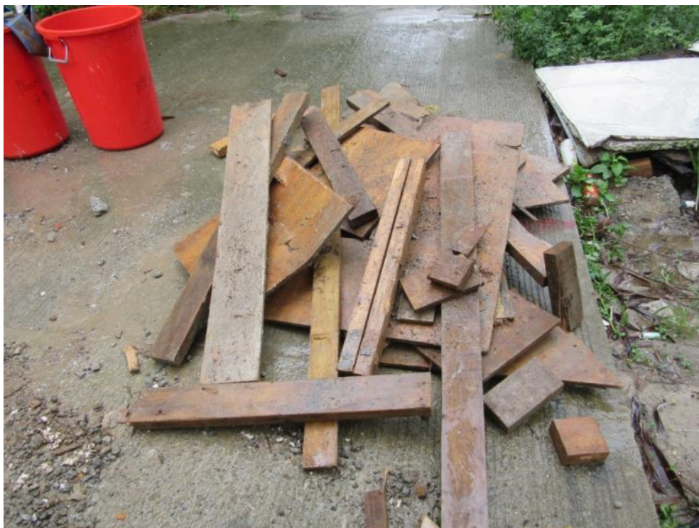
Photo A30: Major Construction Waste from Site C (II)
