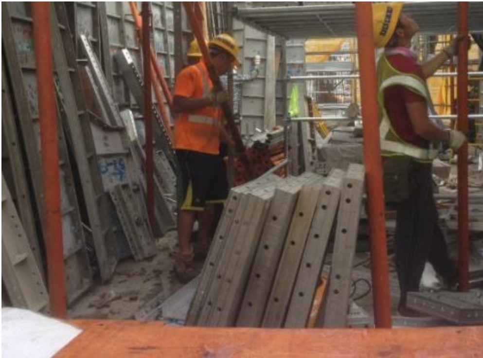
Photo 74: Installing of Aluminium Formwork (1)
