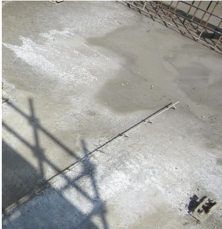
Photo 49: Completion of Concreting
