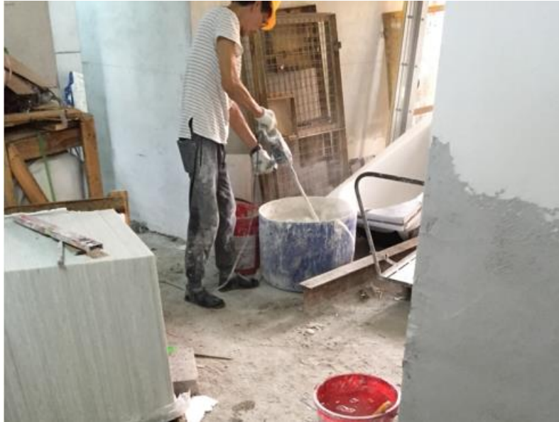
Photo 9: Application of Sealing Primer
