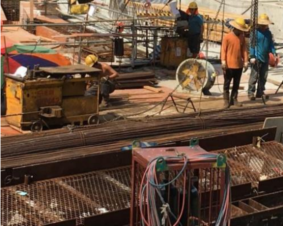
Photo 72: Preparation of Reinforcement Bars
