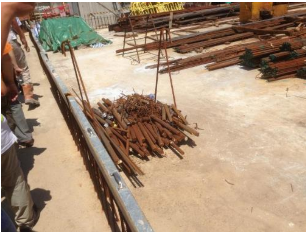
Photo 95: Reinforcement Scraps Sorted for Recycling (1)
