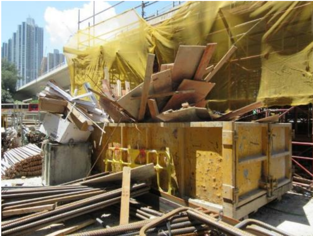
Photo 65: Storing Construction Waste in Skip B
