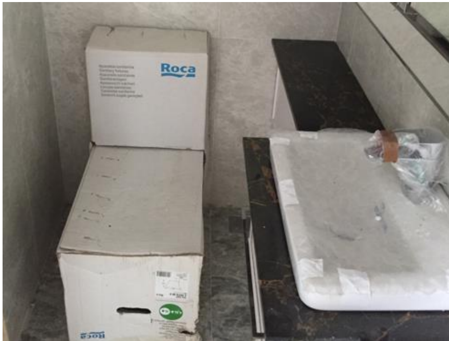
Photo 4: Sanitary Fittings in Bathroom (1)
