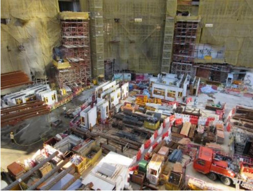
Photo 59: Specific Construction Material Temporary Storage Space
