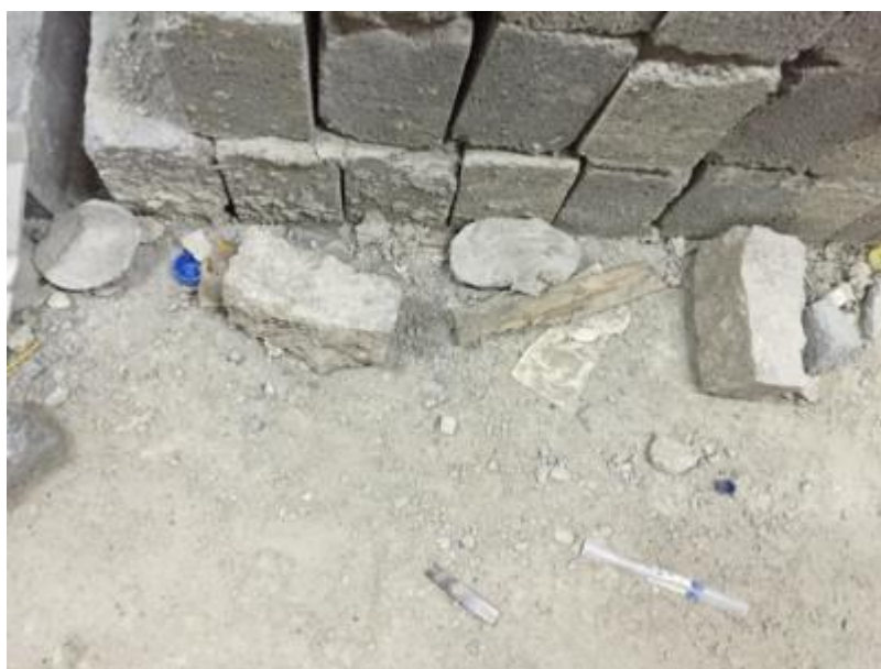
Photo 14: Broken Bricks at a Brickwork Working Area
