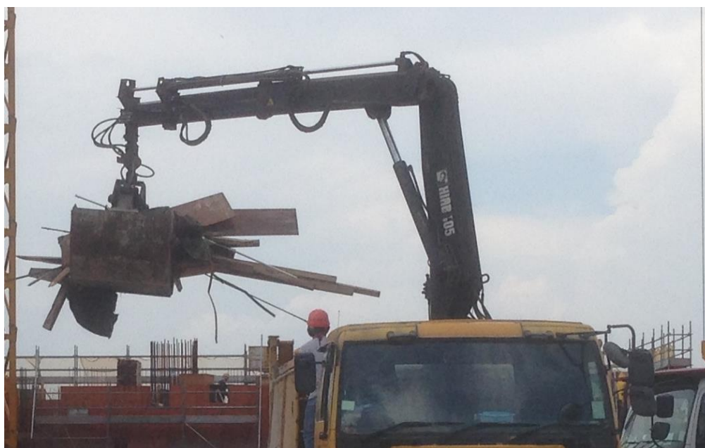
Photo 94: Removal of Construction Waste by Grab Mounted Lorry (2)
