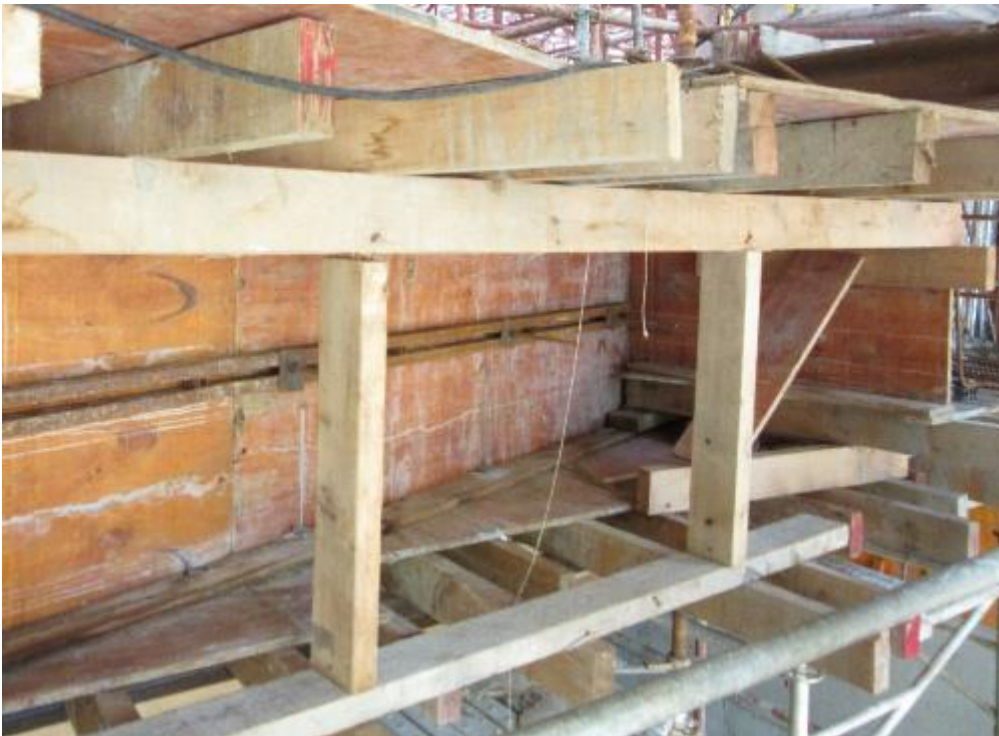
Photo 40: Timber Formwork for Beam of Low-Rise Buildings (1)
