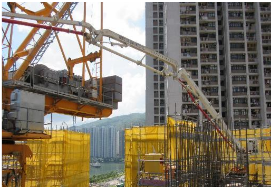
Photo 46: Concreting by Pumping
