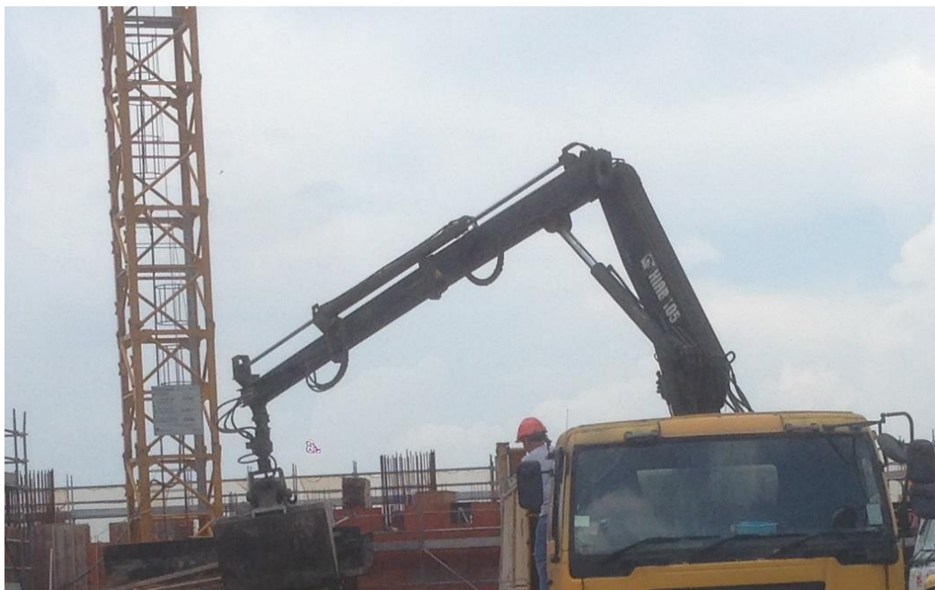
Photo 93: Removal of Construction Waste by Grab Mounted Lorry (1)
