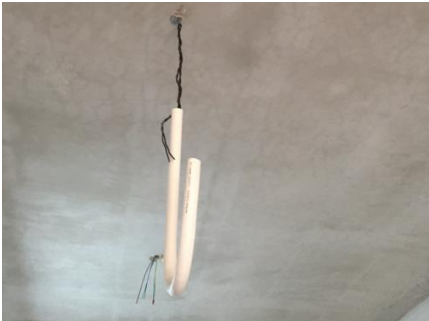
Photo 2: Electrical Connection Setting (2)
