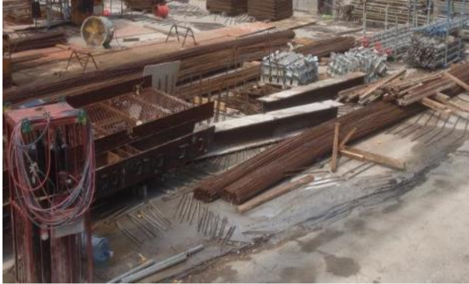
Photo 87: Specific Construction Material Temporary Storage Space
