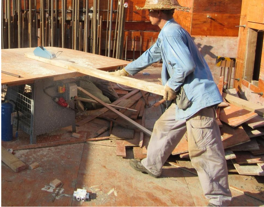
Photo 43: Cutting Timber on Site
