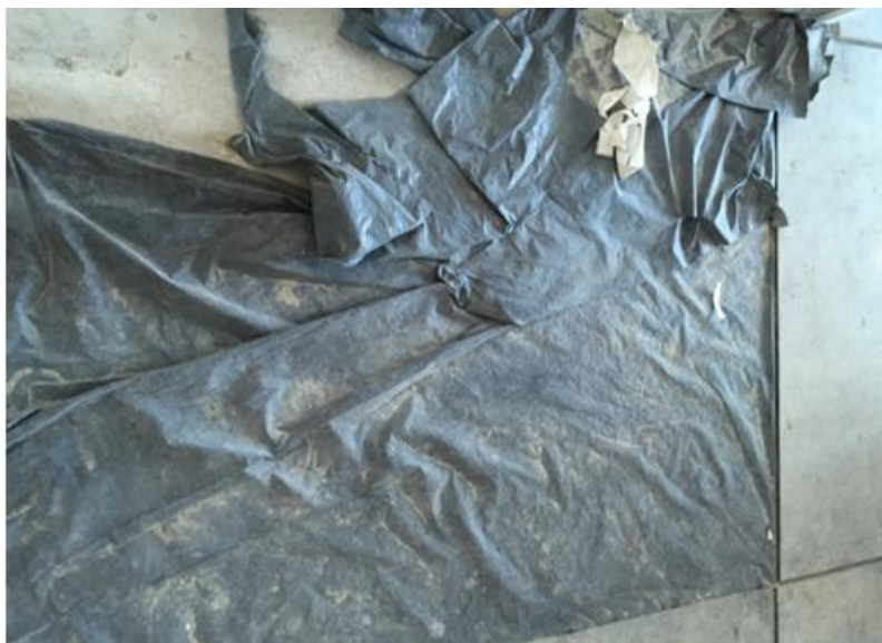
Photo 13: Protection to New Tiled Wall
