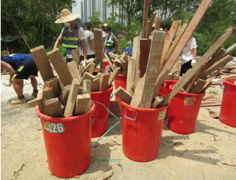
Photo A25: Major Construction Waste from Site B (I)
