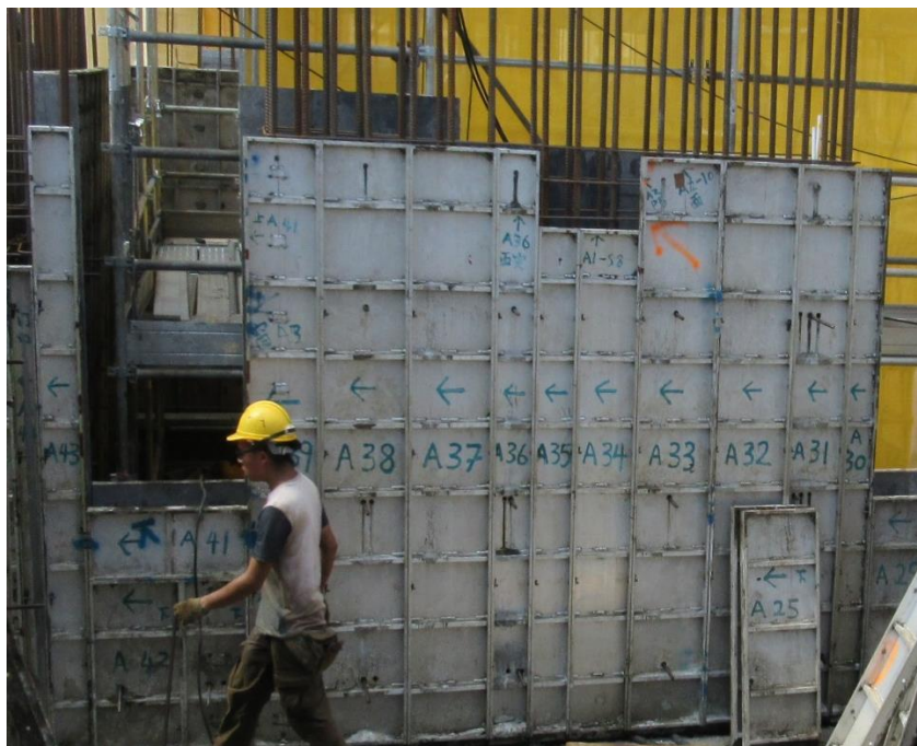
Photo 45: Aluminium System Formwork (2)
