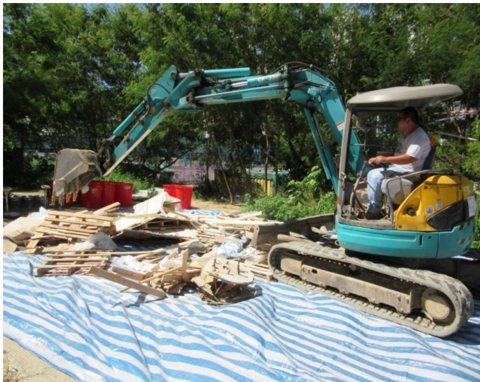
Photo A7: Using Backhoe to Even the Debris (I)
