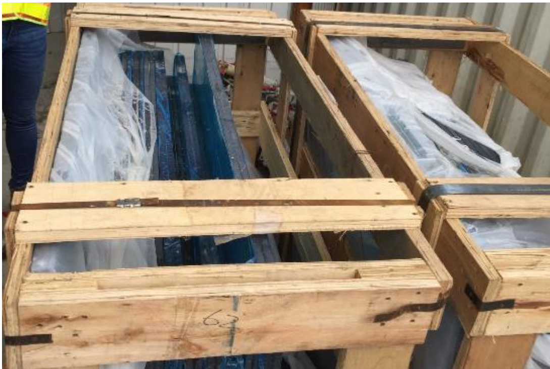
Photo 35: Using Curtain Wall for Building Façade
