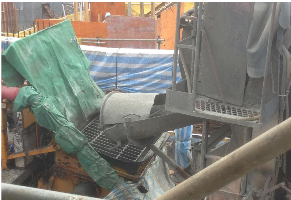
Photo 77: Pouring Concrete to the Pumping Machine
