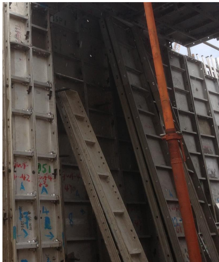
Photo 75: Installing of Aluminium Formwork (2)
