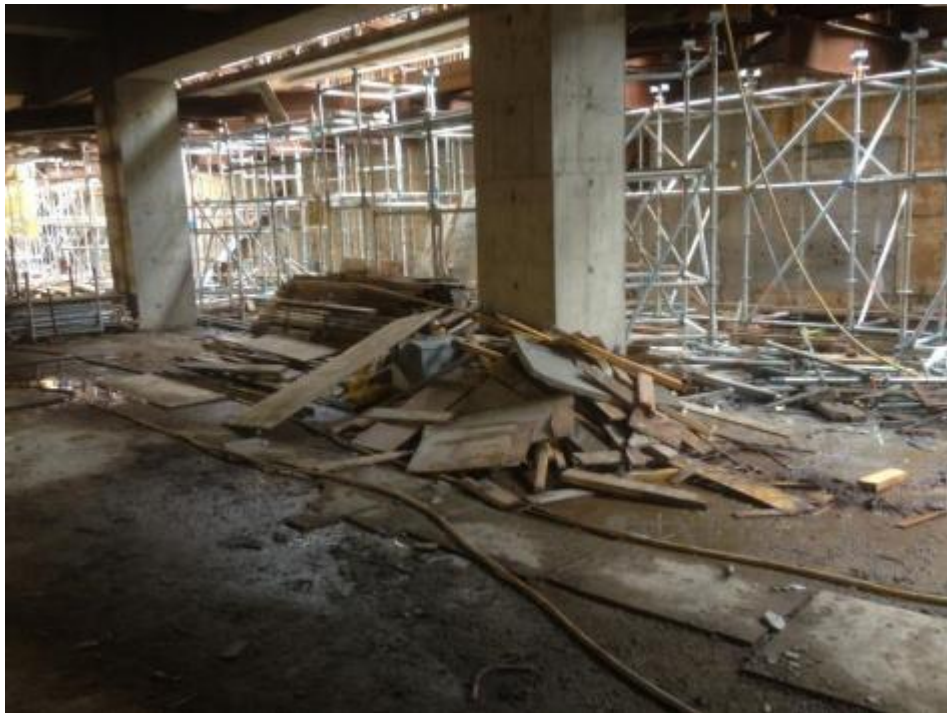
Photo 80: Timber Waste after Removal of Timber Formwork (1)
