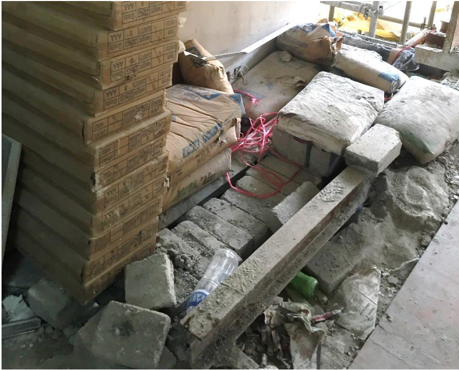
Photo 7: Materials Ready for Brickwork and Tiling
