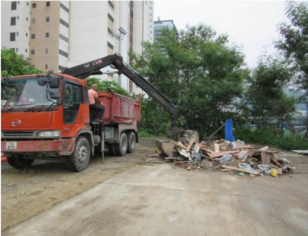
Photo A33: Clearing Construction Waste after Sorting (I)
