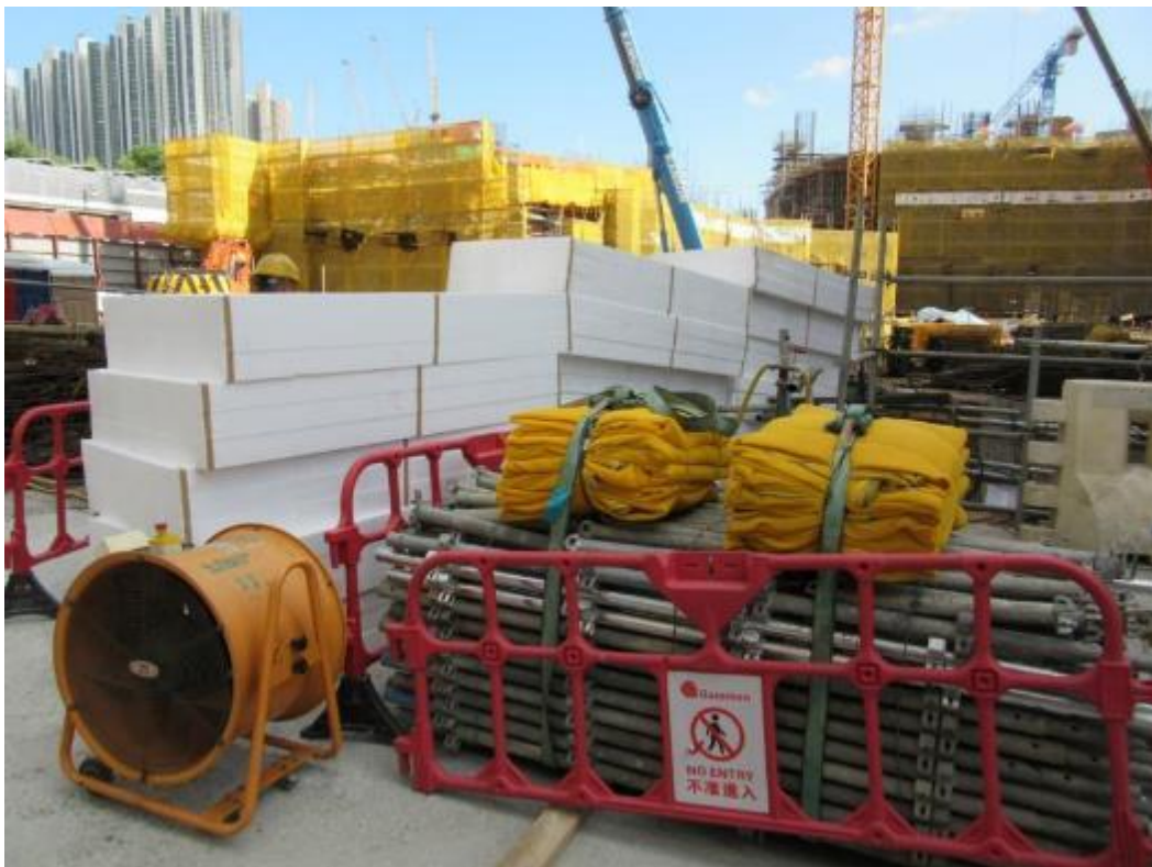
Photo 60: Metal Scaffold Temporary Storage
