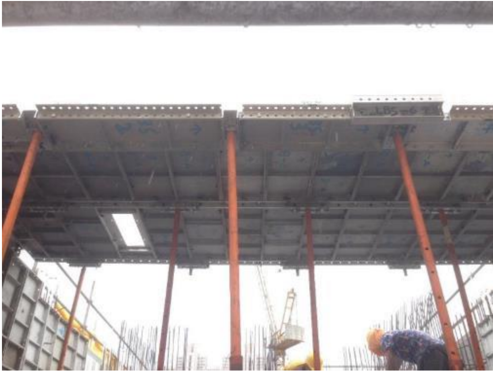
Photo 76: Installation of Aluminium Formwork (3)
