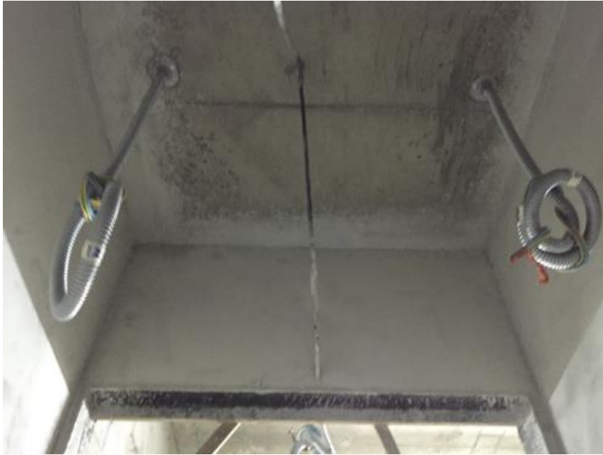
Photo 1: Electrical Connection Setting (1)
