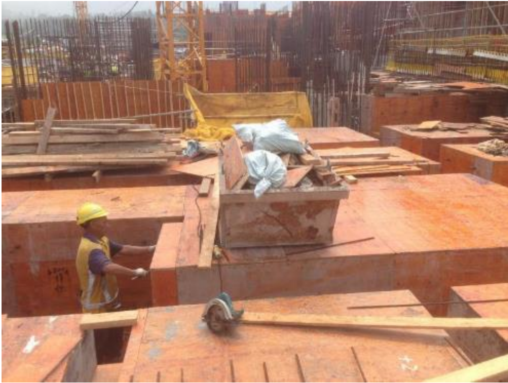
Photo 89: Small Skip for Collecting Waste at the Working Area (1)
