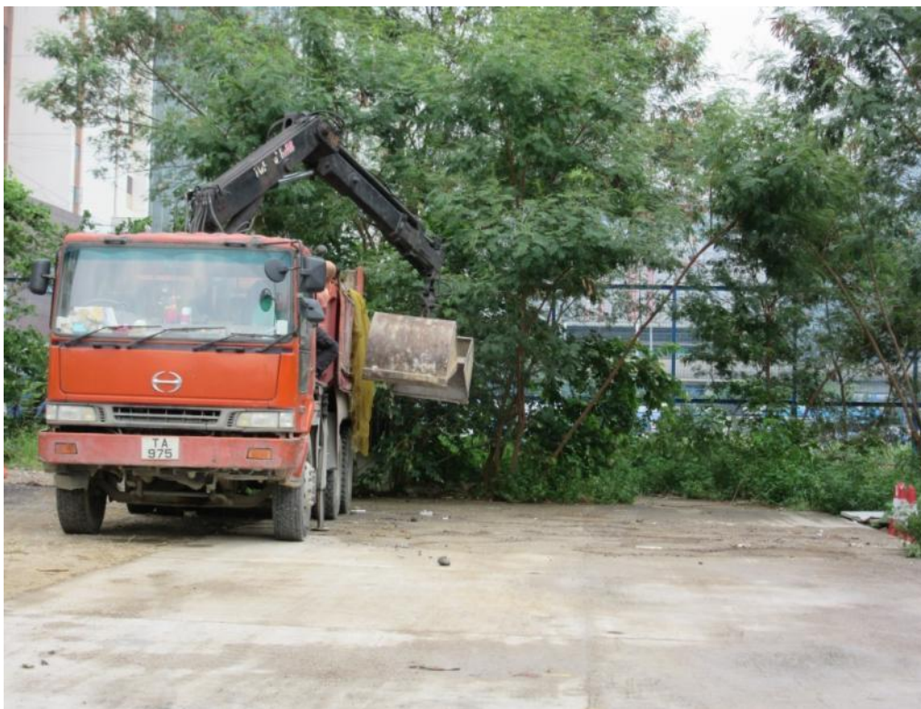
Photo A34: Clearing Construction Waste after Sorting (II)
