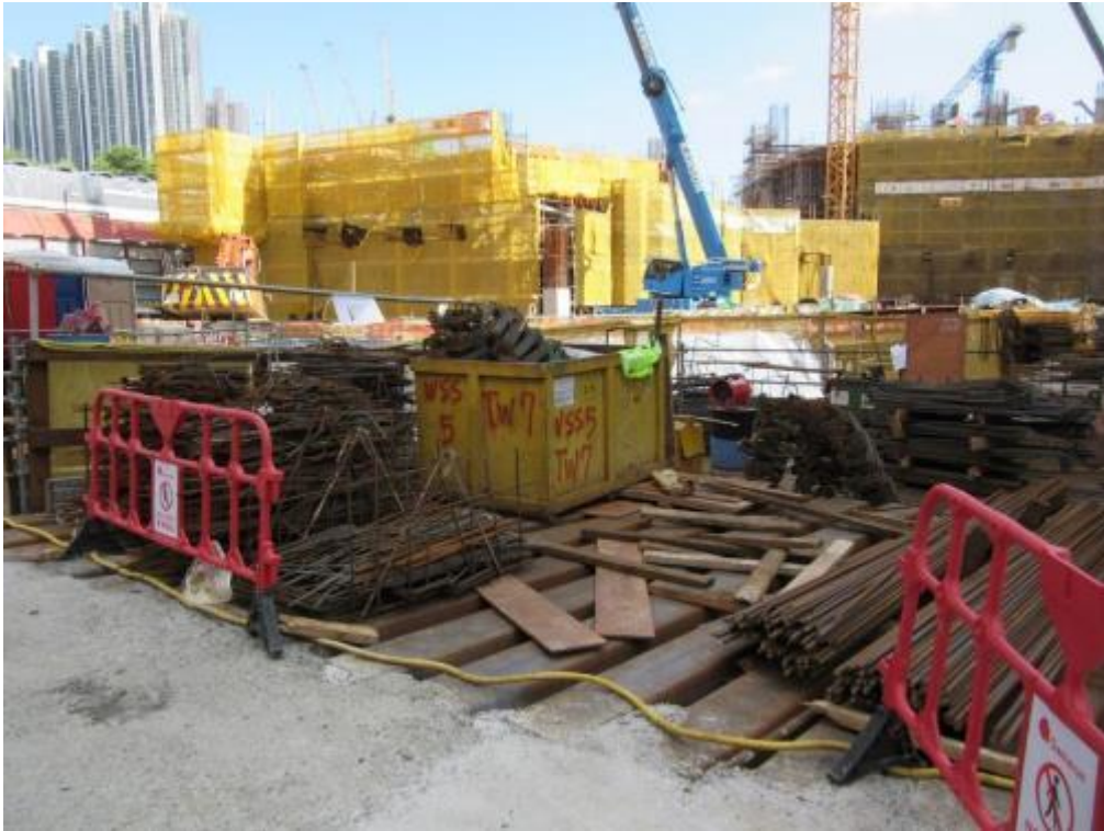
Photo 61: Temporary Storage for Reinforcement Bars
