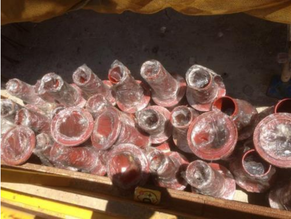
Photo 99: Plastic Packaging of Aluminium System Formwork for Reuse
