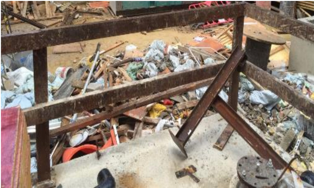
Photo 29: Third Temporary Dumping Location (Area C)
