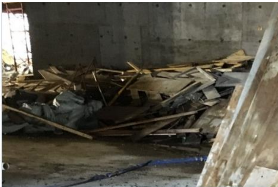
Photo 81: Timber Waste after Removal of Timber Formwork (2)
