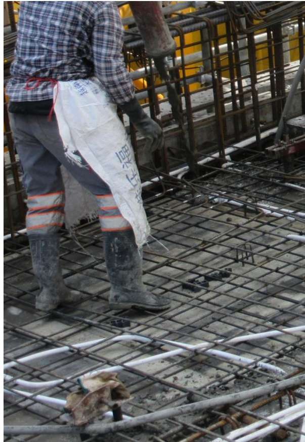
Photo 47: Concreting – in Progress
