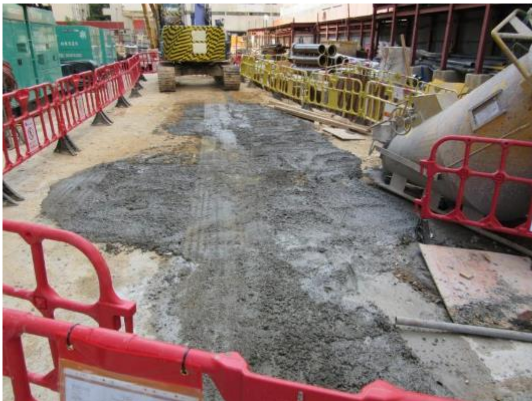
Photo 68: Surplus Concrete for Paving Temporary Access
