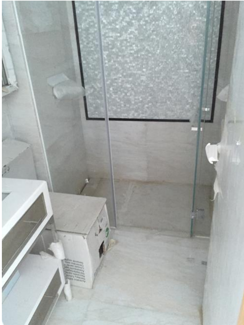
Photo 5: Sanitary Fittings in Bathroom (2)
