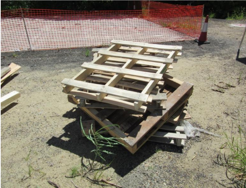
Photo A21: Major Construction Waste from Site A (I)
