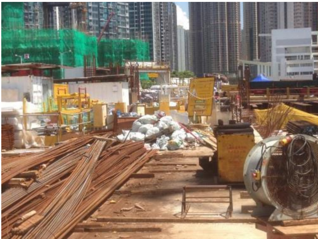
Photo 92: Dedicated Location for Collecting Construction Waste
