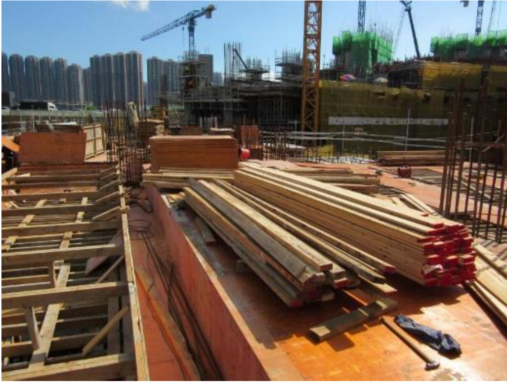
Photo 39: Timber Formwork for Decking of Low-Rise Buildings
