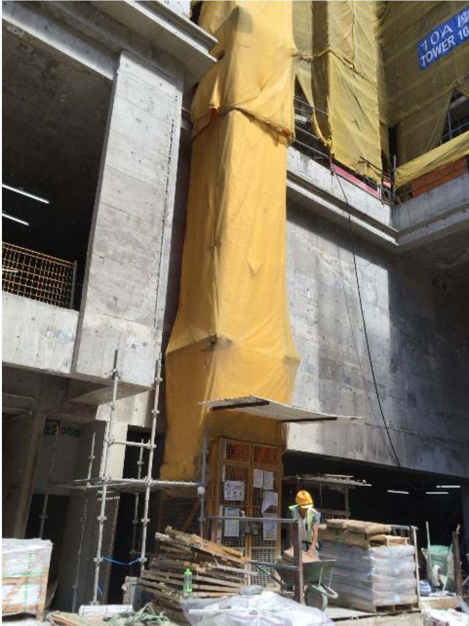
Photo 36: Use of Refuse Chute to Transport Construction Waste from Building
