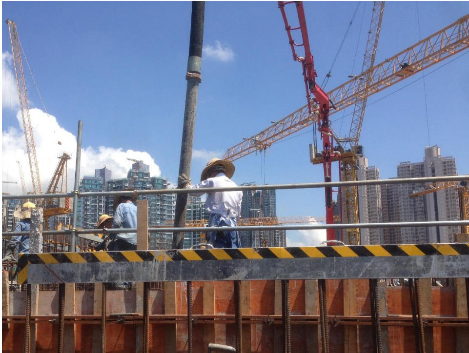
Photo 79: Concreting by Pumping
