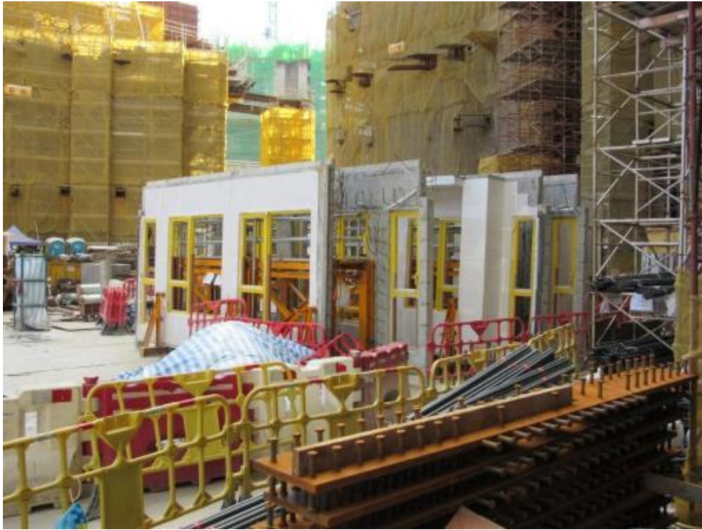
Photo 63: Use of Precast Units
