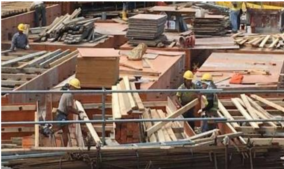
Photo 73: Timber Formworking
