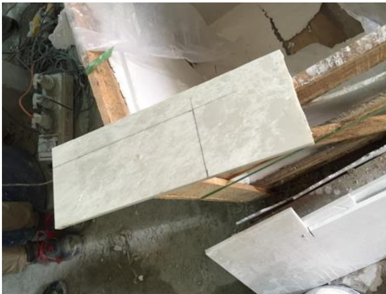
Photo 10: Planning/Measurement before Tile Cutting
