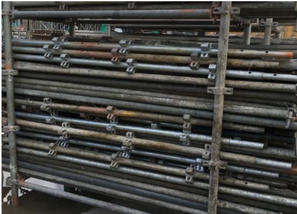
Photo 88: Metal Scaffold Temporary Storage
