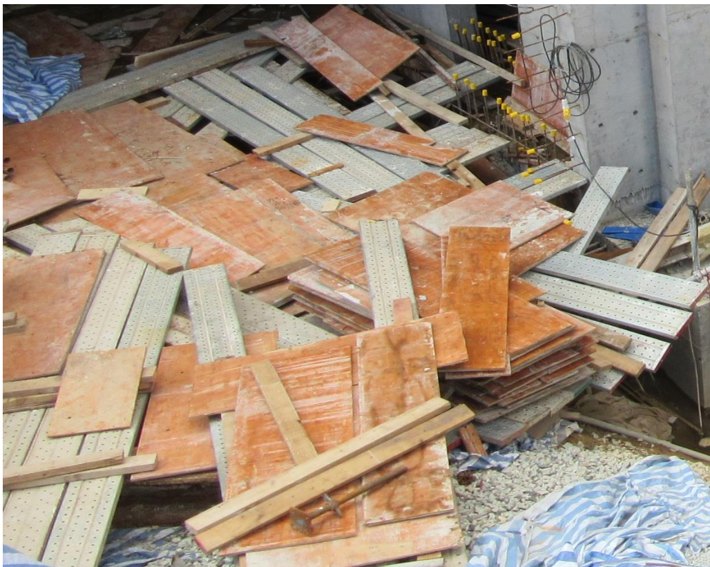
Photo 54: Used Timber to be sorted after Removal of Timber Formwork
