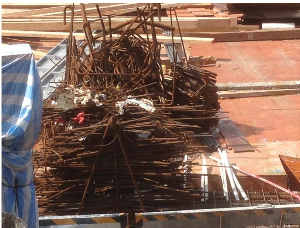
Photo 96: Reinforcement Scraps Sorted for Recycling (2)
