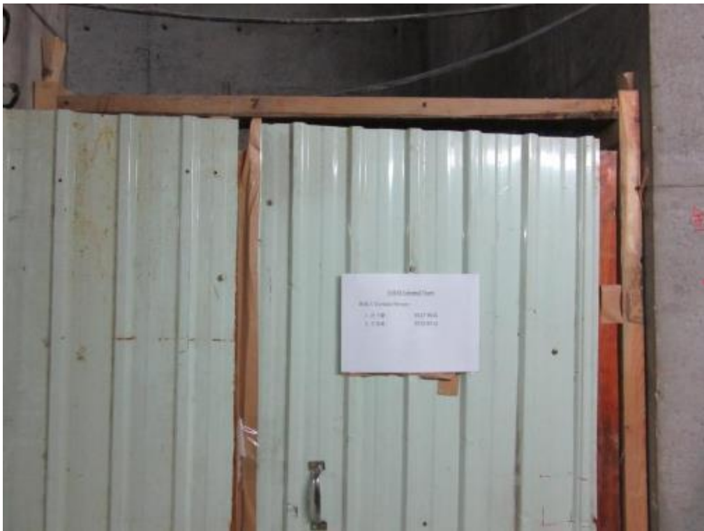
Photo 70: Reuse of Scraped Timber for Frame of Temporary Door
