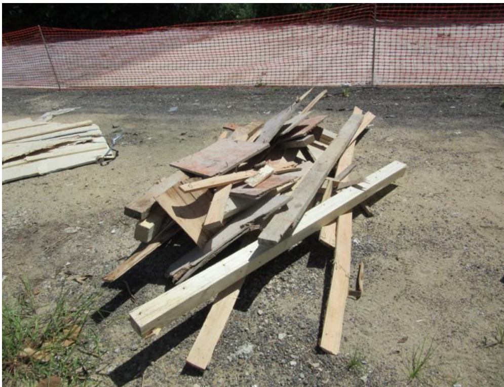
Photo A22: Major Construction Waste from Site A (II)
