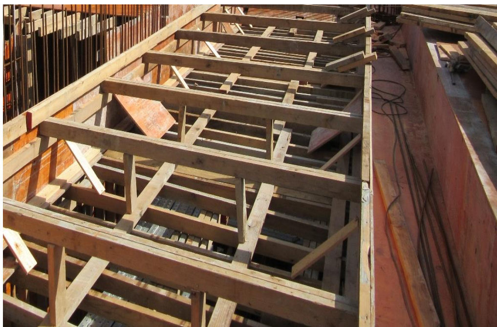
Photo 41: Timber Formwork for Beam of Low-Rise Buildings (2)
