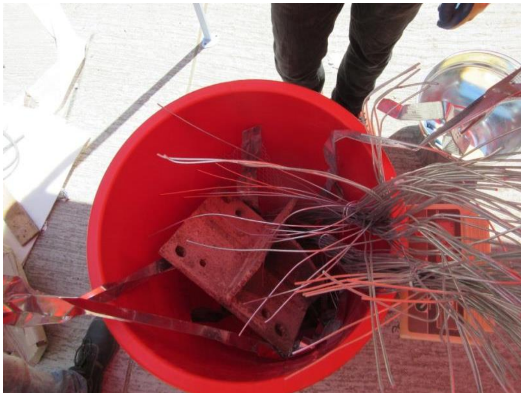
Photo A23: Some Other Construction Waste from Site A (I)
