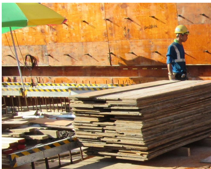
Photo 42: Preparation Area of Timber Formwork
