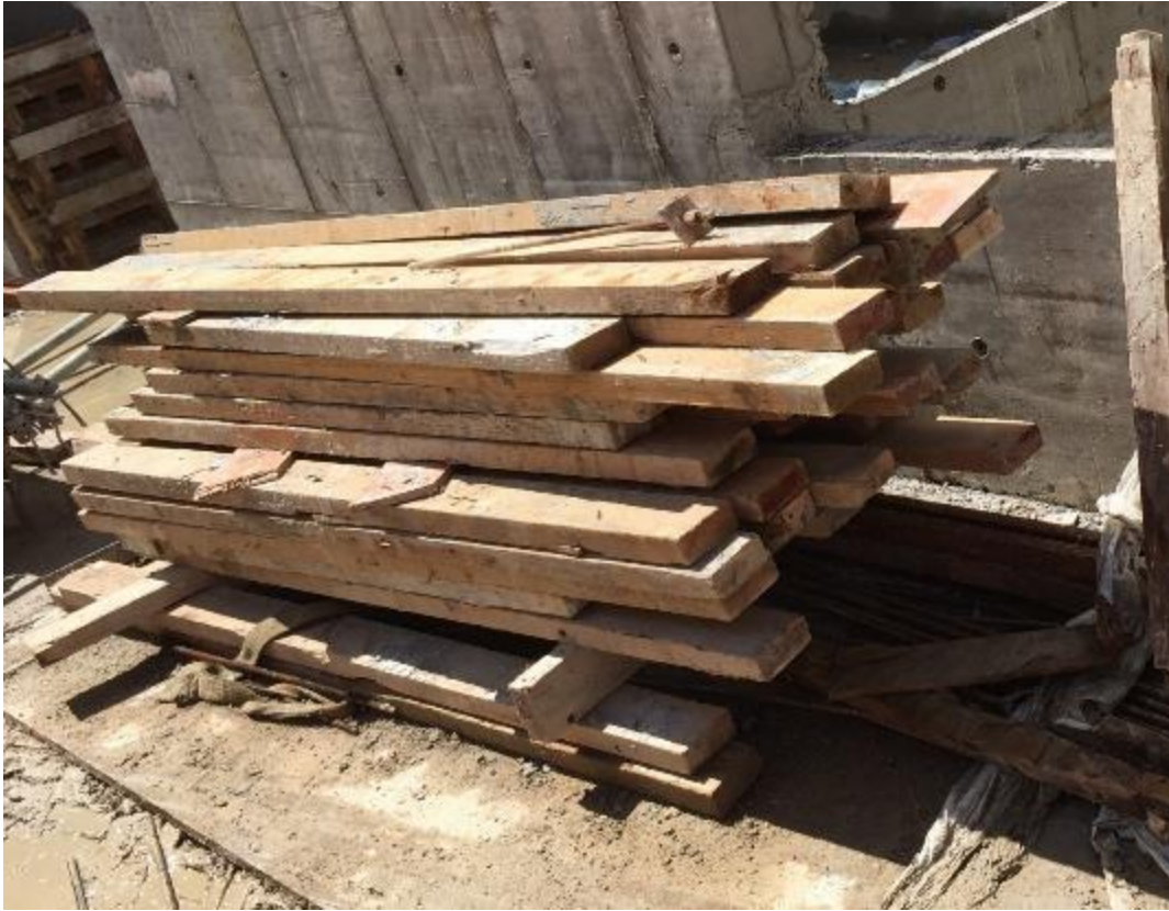
Photo 34: Ends of Timber and Metal Channels to be Reused
