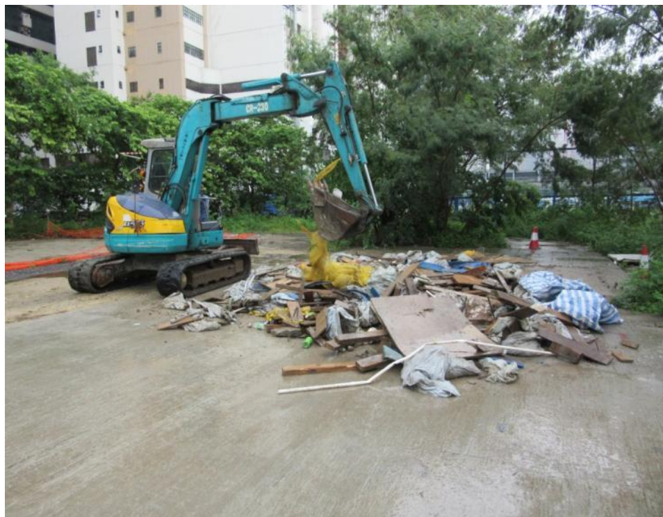
Photo A8: Using Backhoe to Even the Debris (II)
