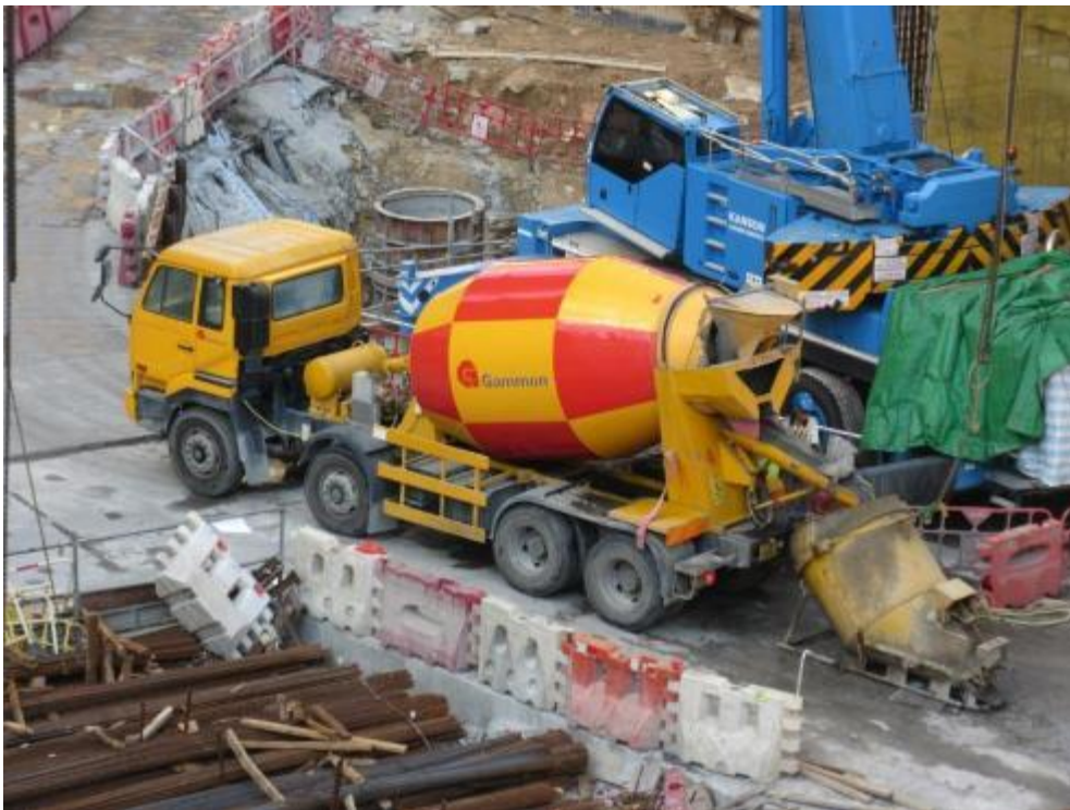
Photo 50: Concreting by “Crane + skip”
