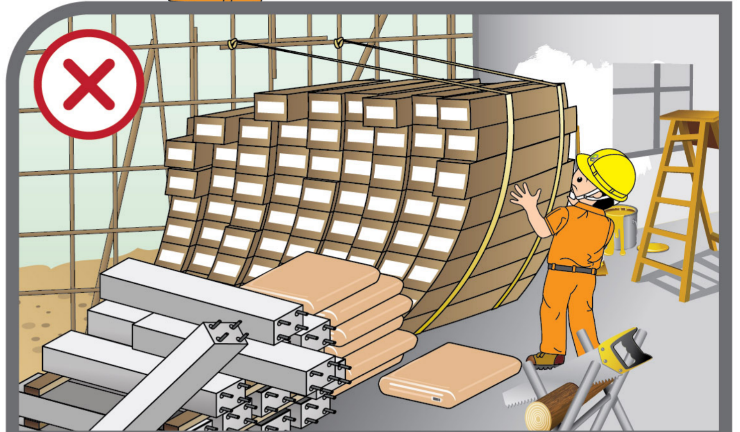
Unsafe stacking and unsafe tying to the scaffolding
