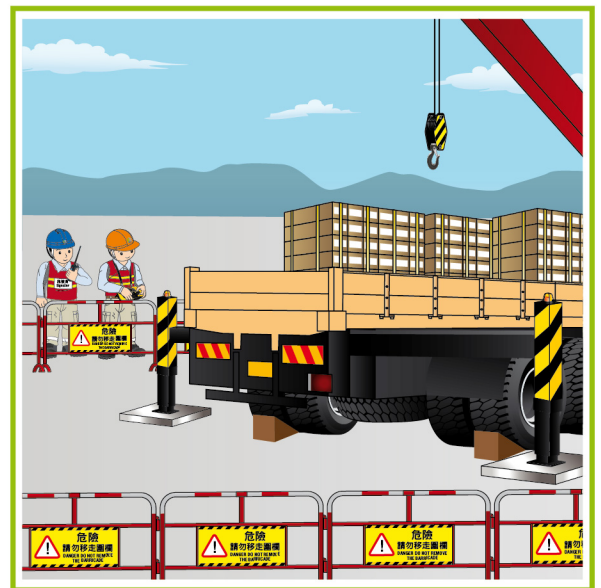
The fatal zone should be barricaded before lifting operation.
